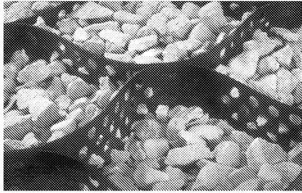
Cellular confinement system filled with angular stone
