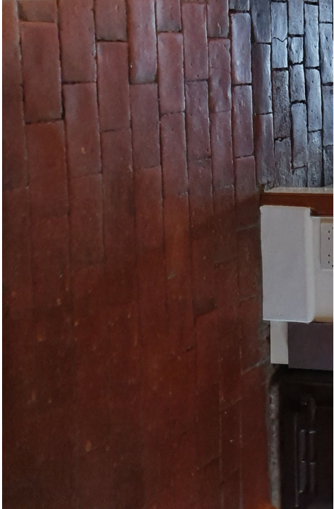
Brick flooring to kitchen
