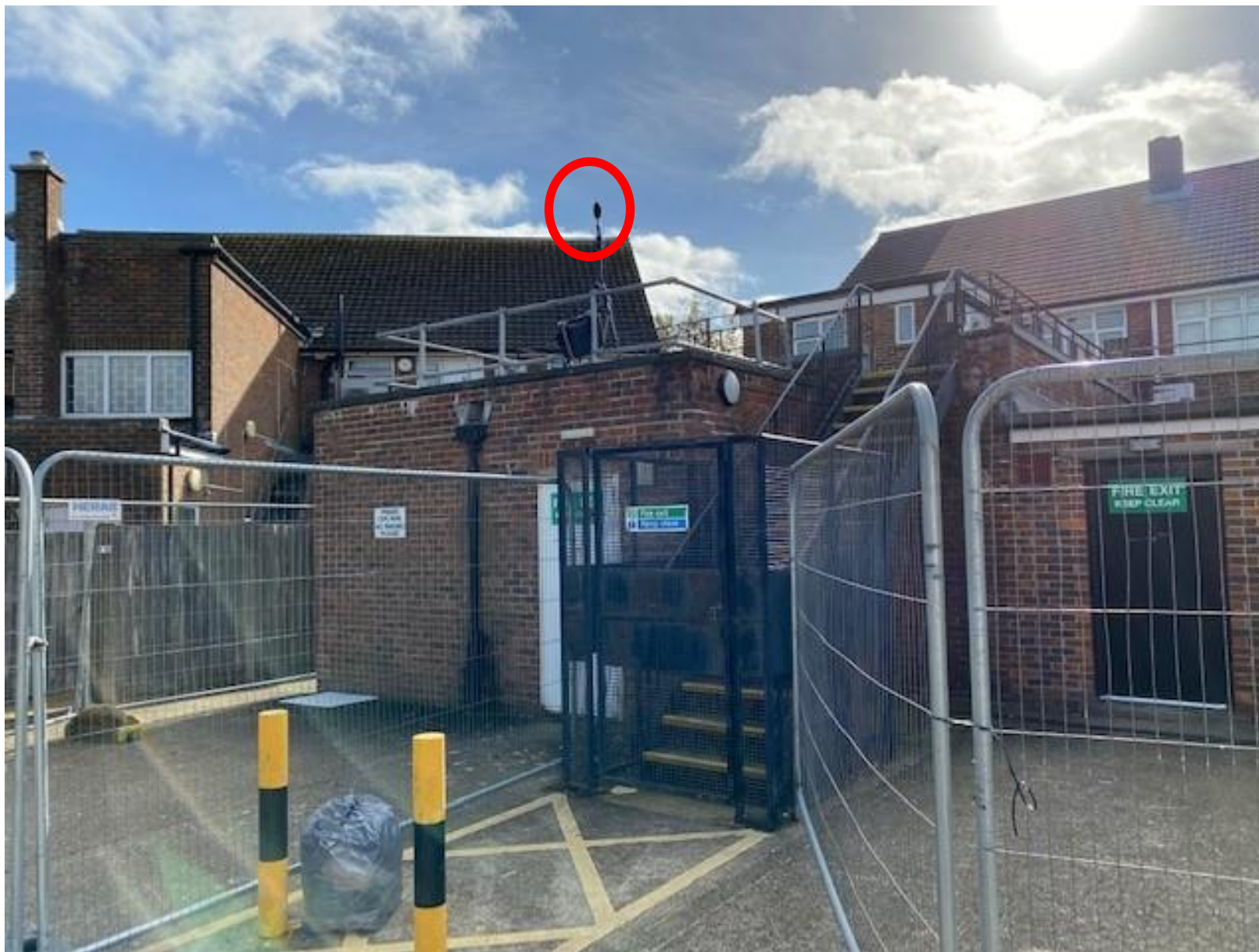
114 – 116 The Street, Littlehampton BN16 3DA Photograph Showing Measurement Position Project 11416
