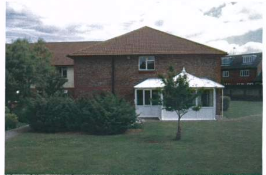
View of the area of proposed extension and the conservatory to be demolished
