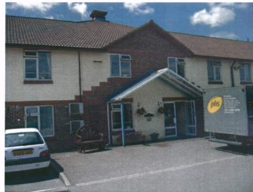
Existing Front Entrance with Level Access
