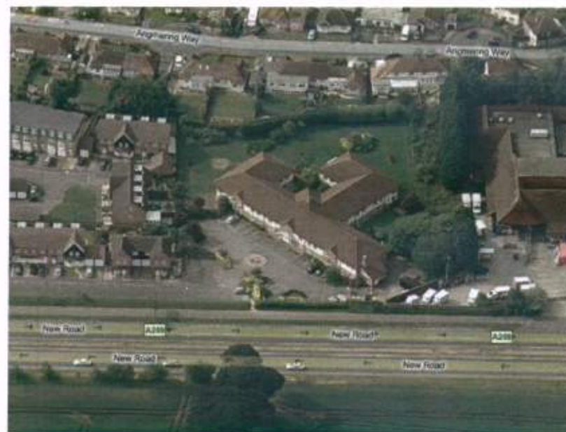
Aerial photo of site
