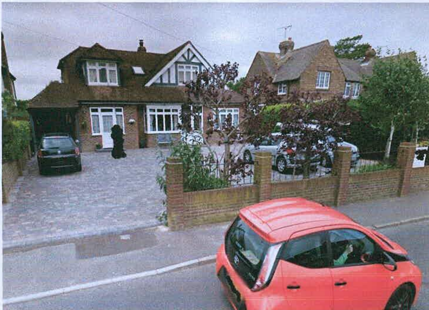
Street view of similar wall in North Lane
