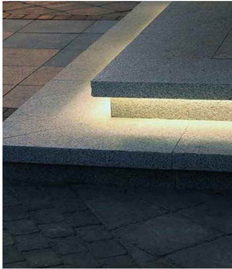
Example of strip lighting to be positioned under timber coping of retaining beds
