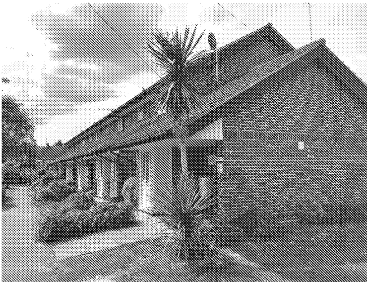
Successful example of existing stepped roof arrangements on apartments 99-101 & 115-117.
