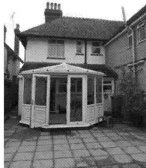
Part of rear elevation – Existing conservatory
