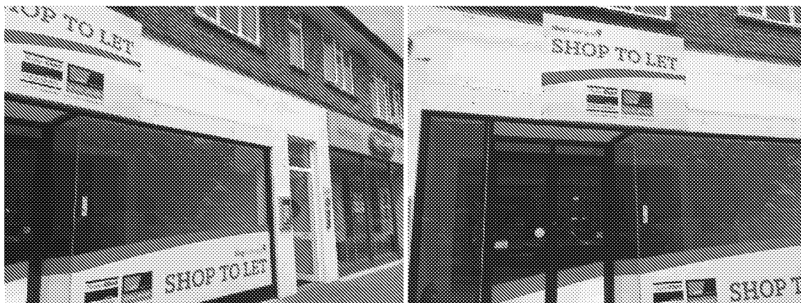
Figures 2.1 and 2.2: The Site – Photographs Taken on Site Visit on 4 th July 2018
