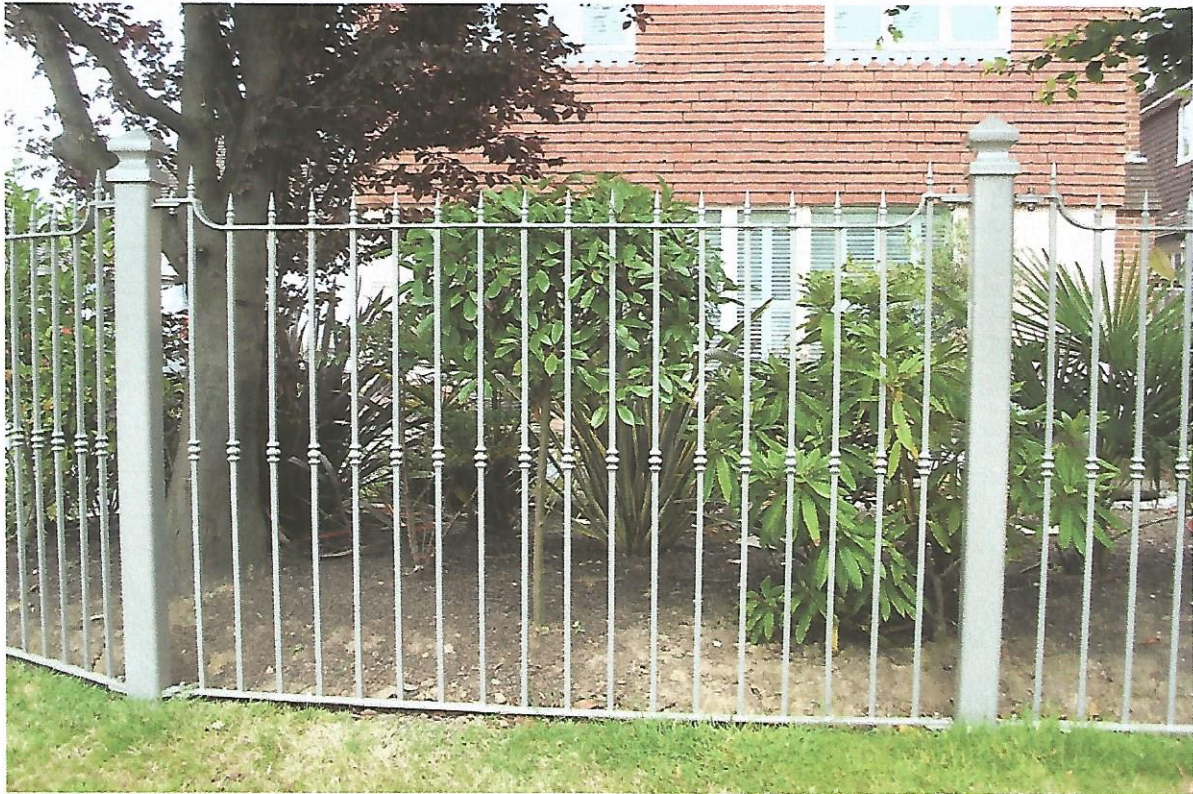
Continuing panel following gates on the east section of the front boundary metal railings.
