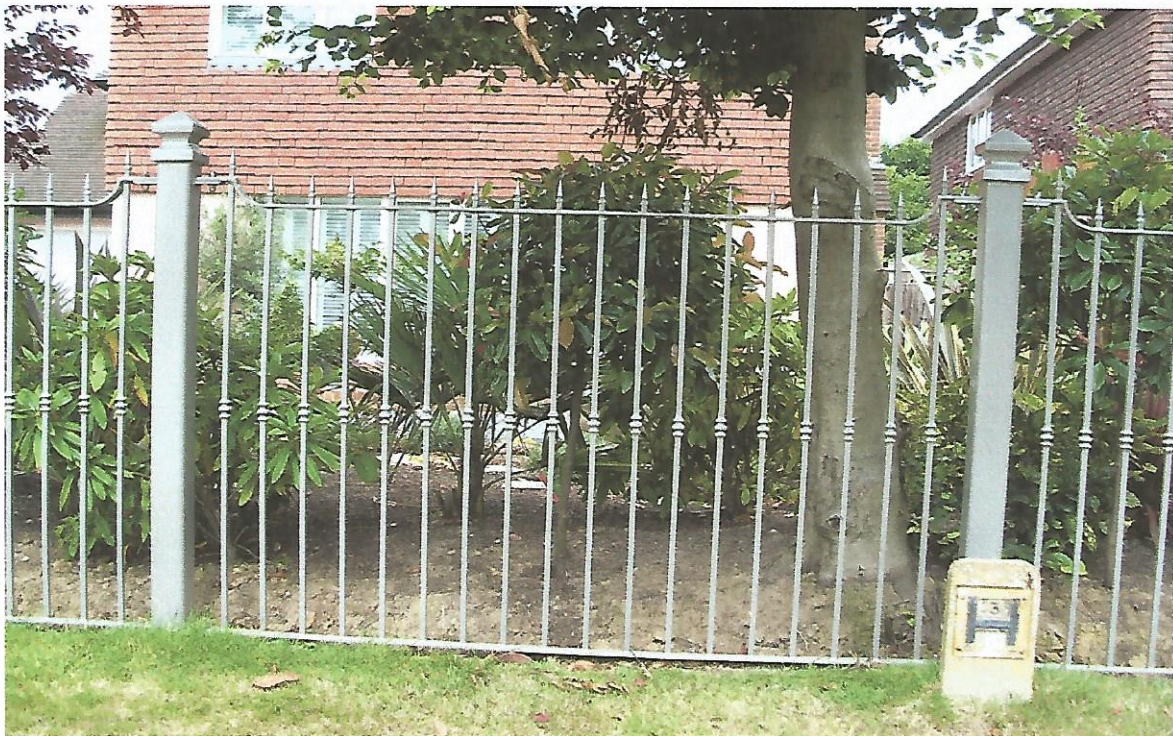
Next panel following gates on the east section of the front boundary metal railings.
