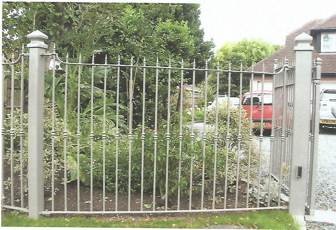
Next panel on west section of front boundary metal railings.
