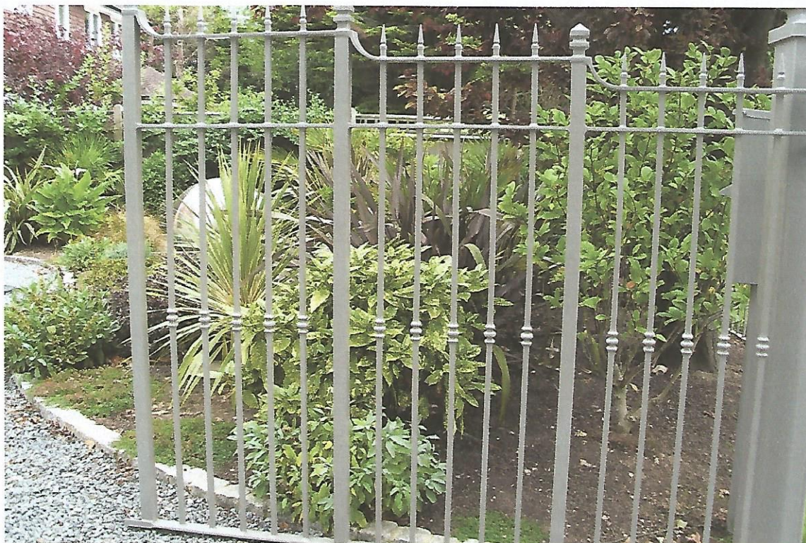
Gates to east section of front boundary metal railings.
