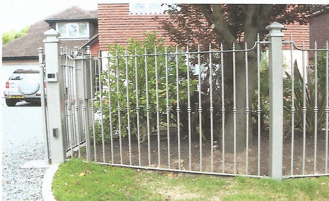
1 st Panel after gates on the east section of the front boundary metal railings.
