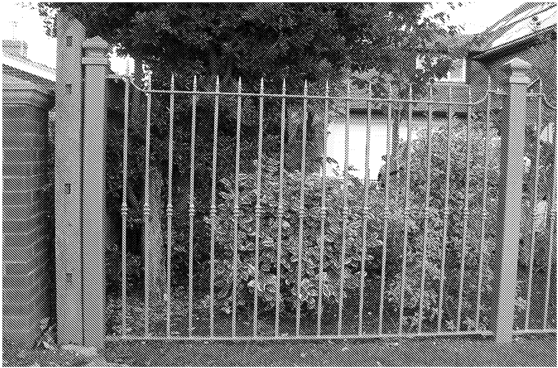
Left (west) hand facing of the front boundary metal railings. 1 st panel.
