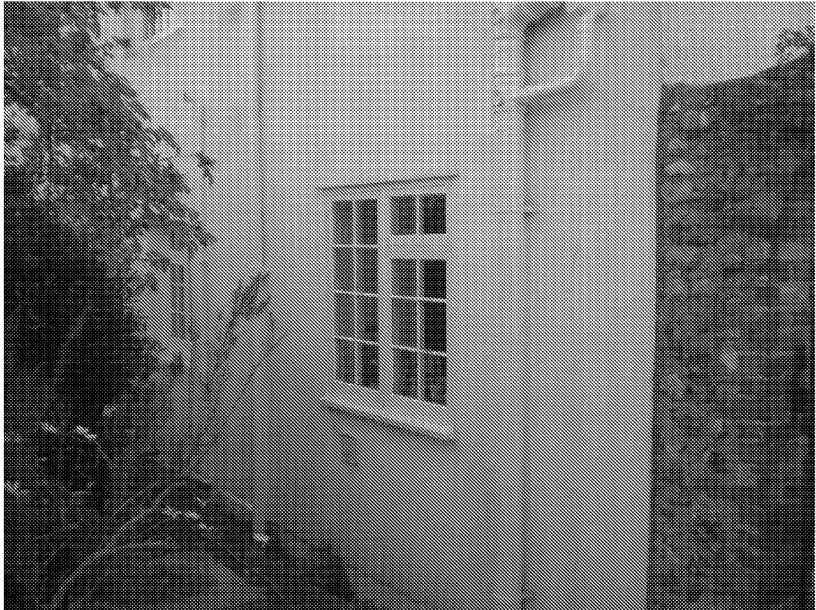
Eastern Elevation: Window GE1
