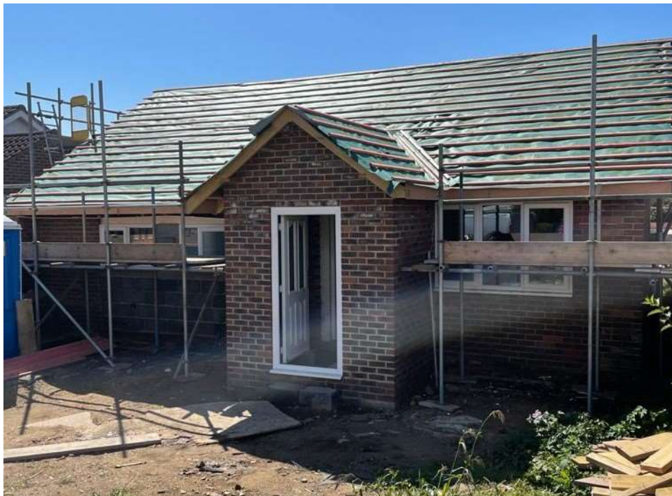
Replacement Porch as Constructed
