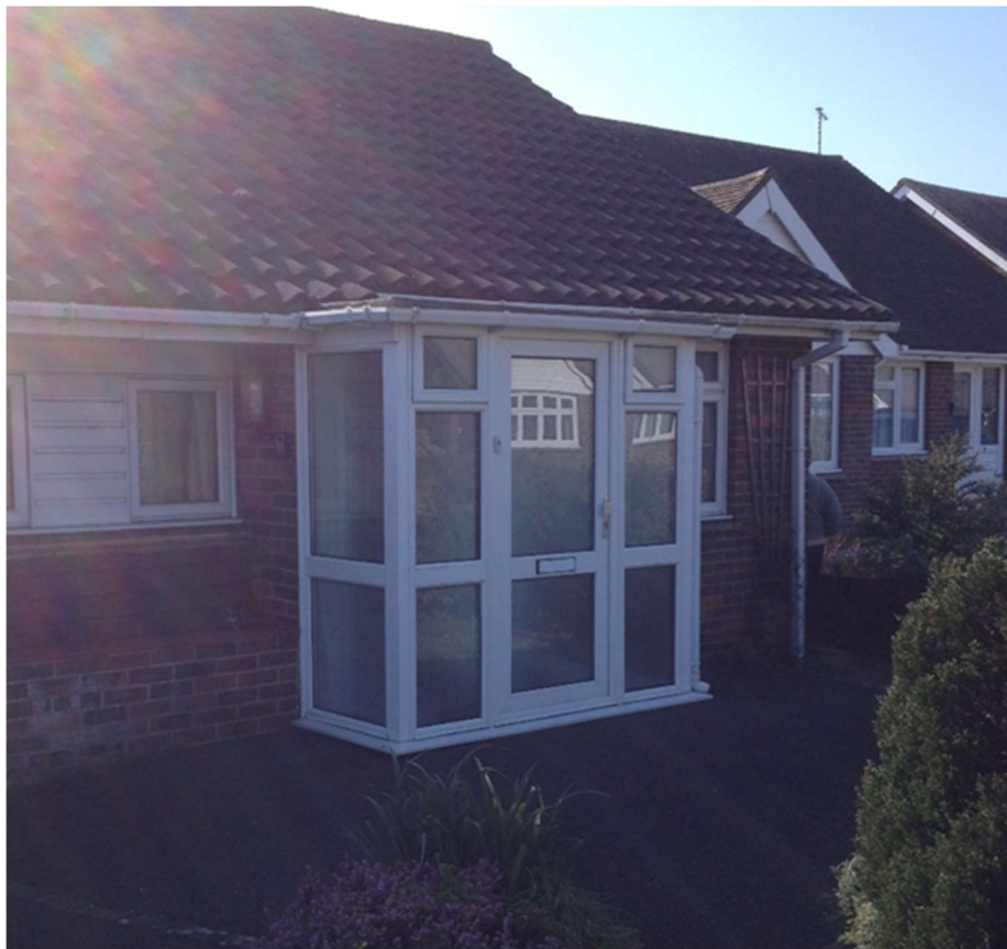
Previous Flat Roofed Porch
