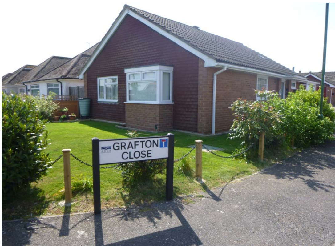
EXISTING FRONT / SIDE VIEW OF PROPERTY
