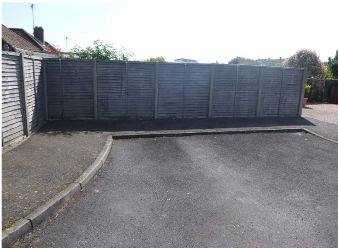
EXISTING REAR SIDE VIEW BOUNDARY TO GARDEN AND GRAFTON CLOSE
