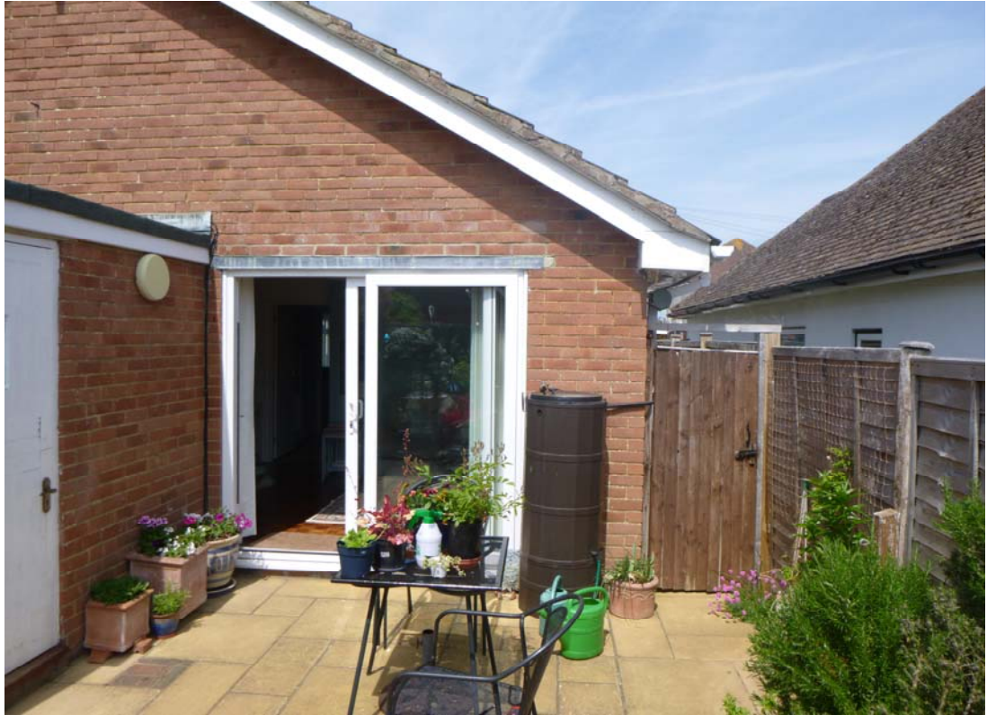
EXISTING BACK VIEW OF PROPERTY
