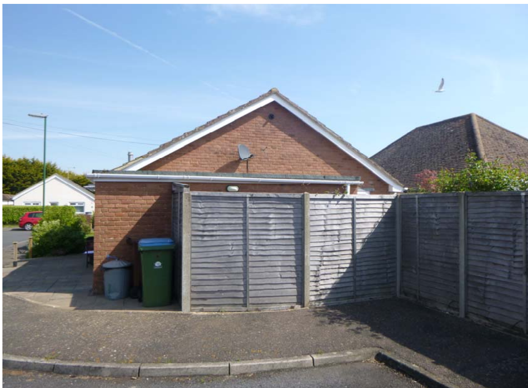
EXISTING REAR VIEW OF PROPERTY FROM GRAFTON CLOSE
