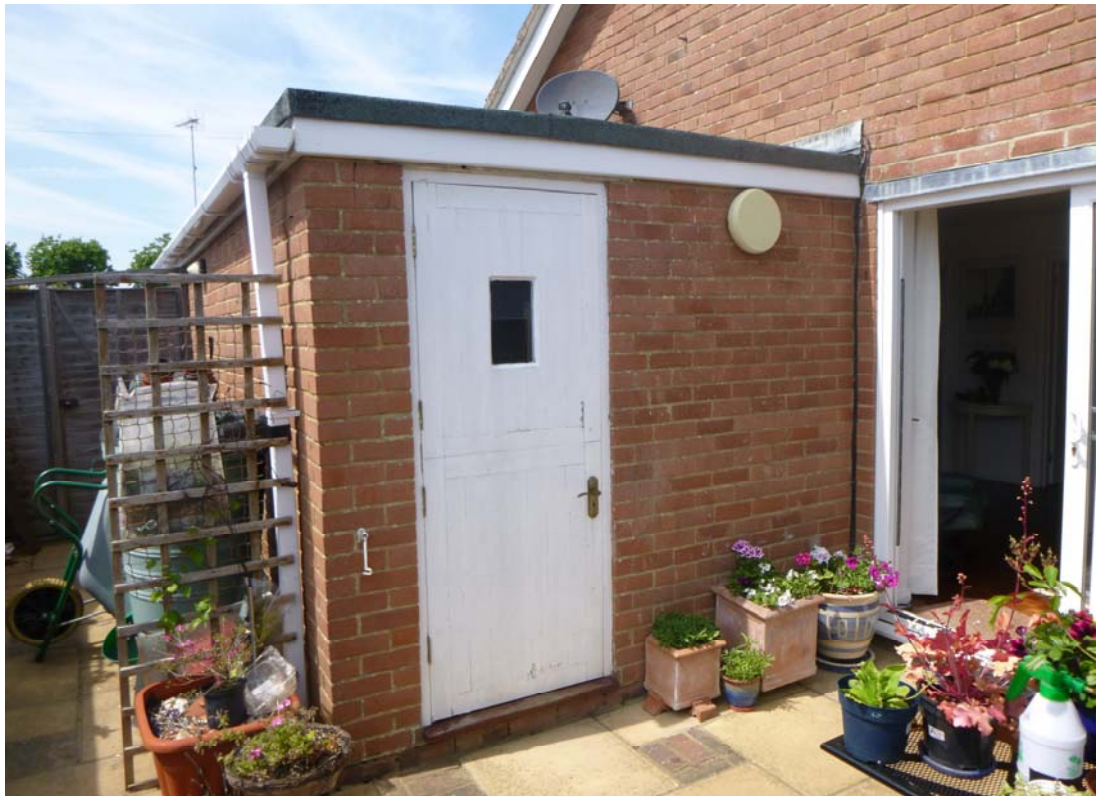
EXISTING BACK VIEW OF GARAGE
