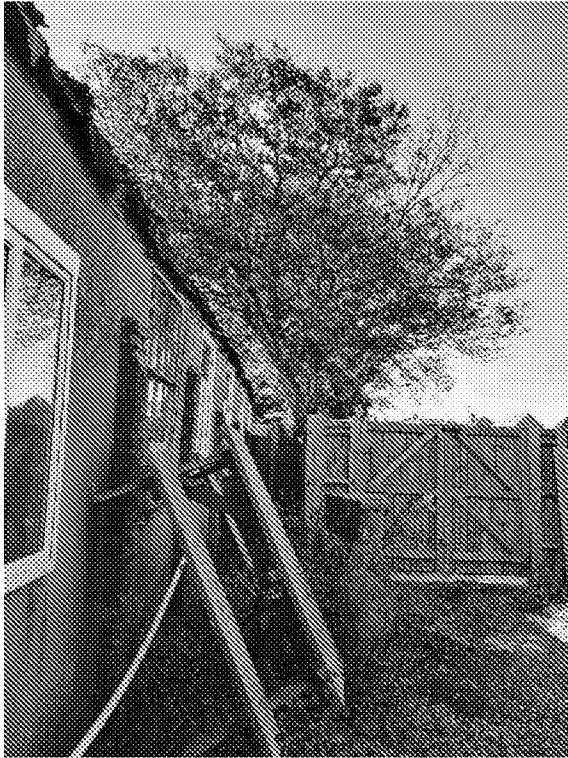
Image 7 External view of Building B2 and adjacent off-site tree.
