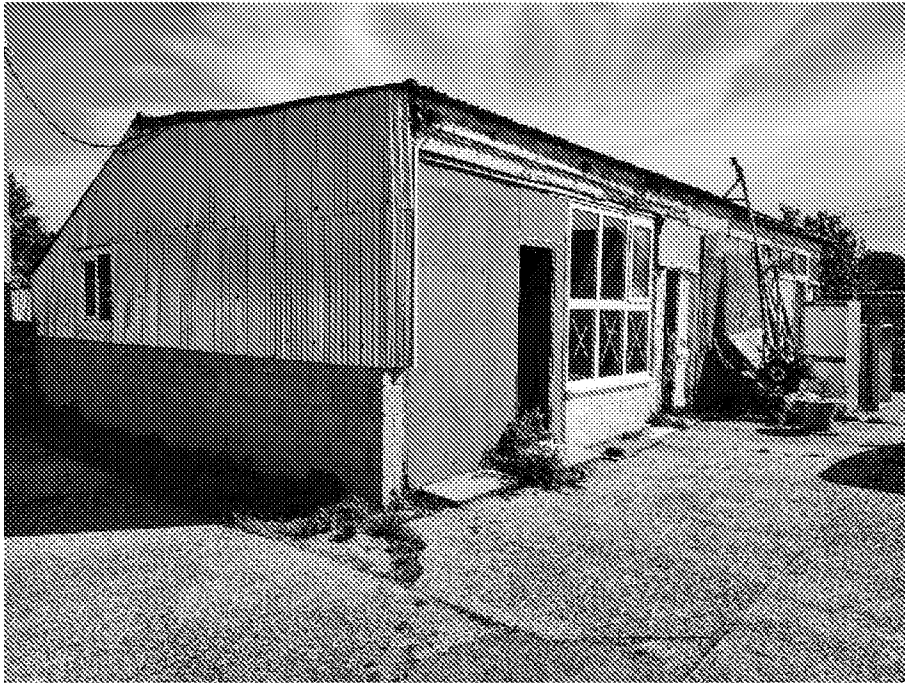
Image 1 External view of Building B1, single story, single skinned structure with high levels of light throughout.
