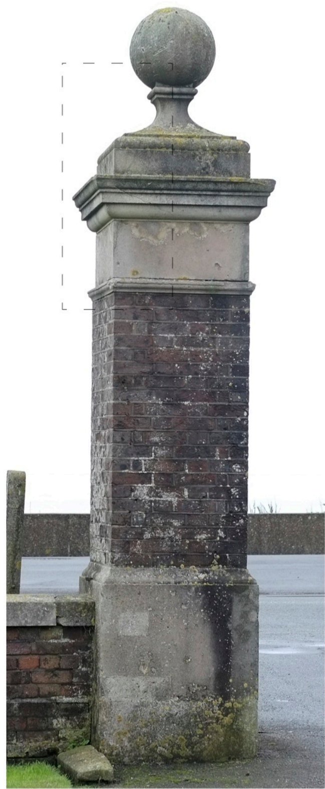
2 Photograph of Existing Pier
