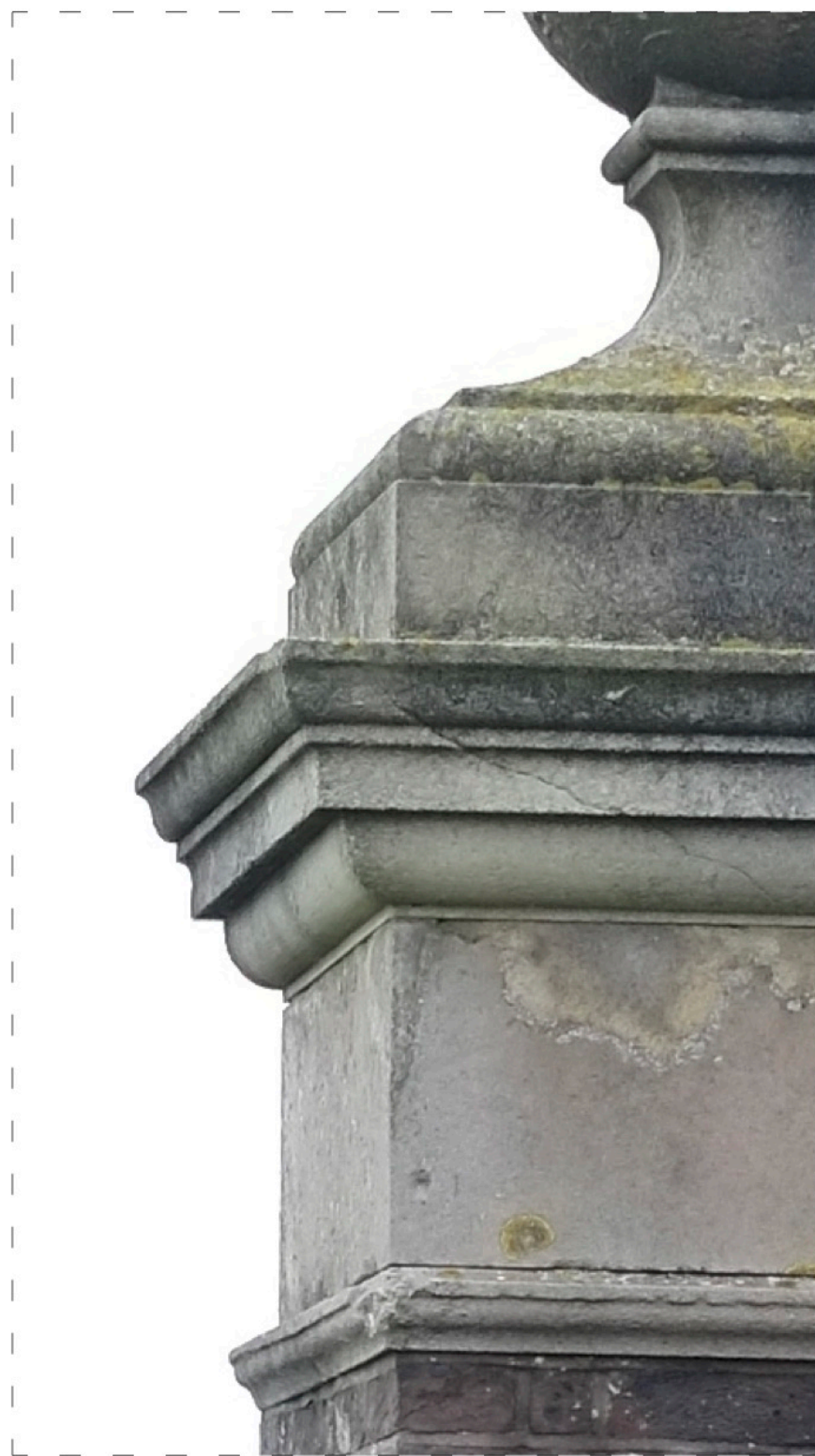
3 Photograph of Existing Pier Detail
