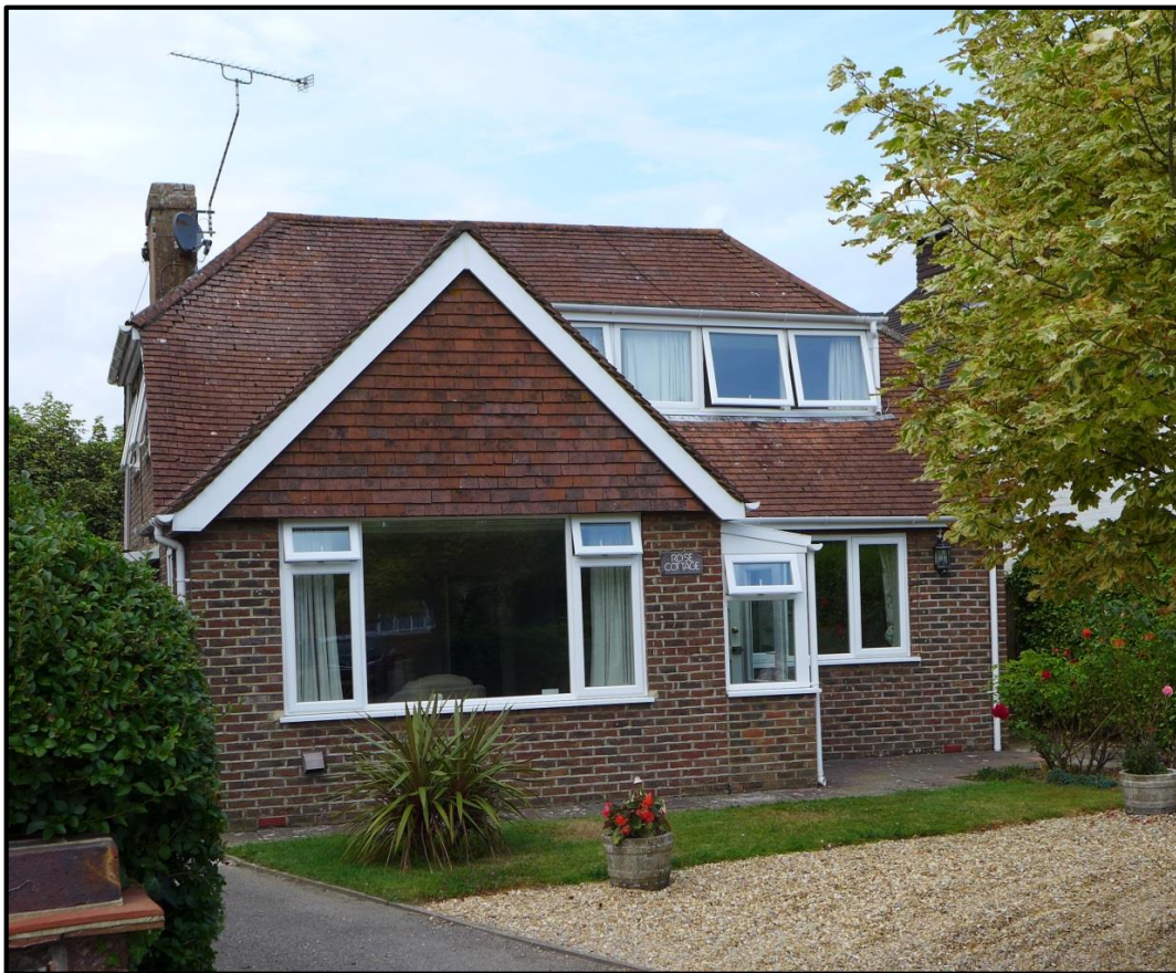
Photograph 1. Rose Cottage, Herne Lane. Chalet style bungalow with barn ended roof to north and south elevations.
