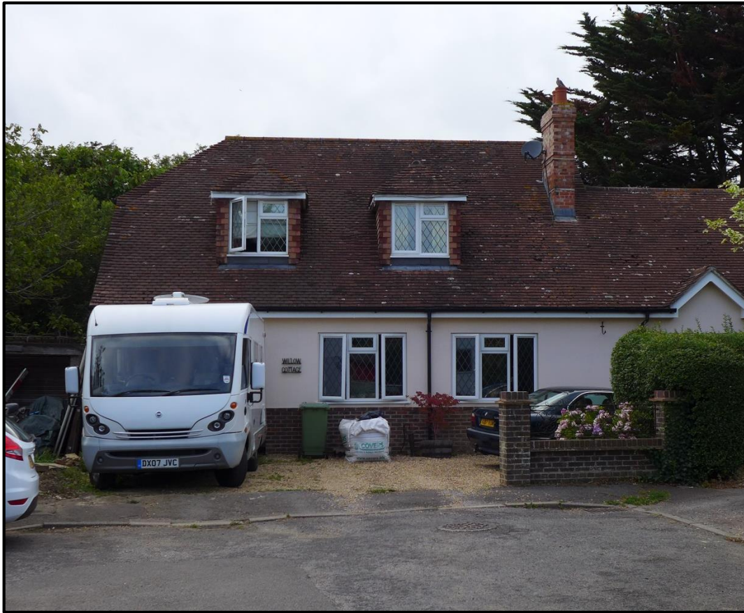
Photograph 2. Willow Cottage, Herne Lane. Narrow pitched roof dormers to front elevation and colourwash render to walls.
