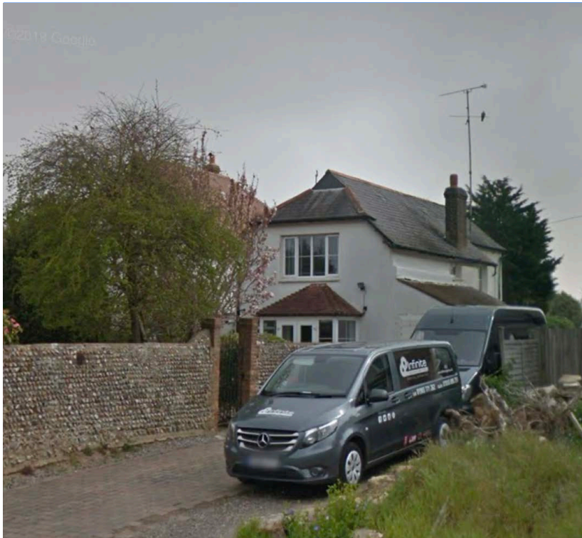
EXISTING HOUSE — VIEW FROM THE STREET
