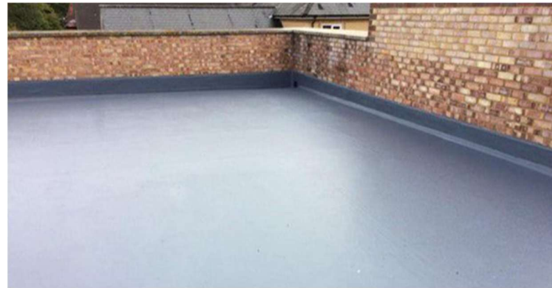
Flat roof finish - Sika sarnafil single roof membrane system
