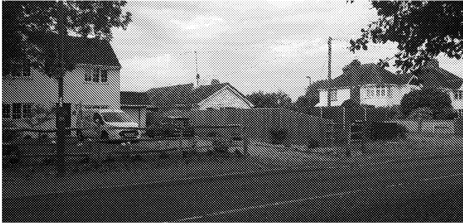
The site in the context of the Mill Lane street scene
