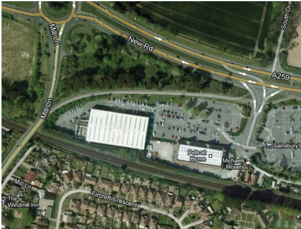
Aerial view of site
