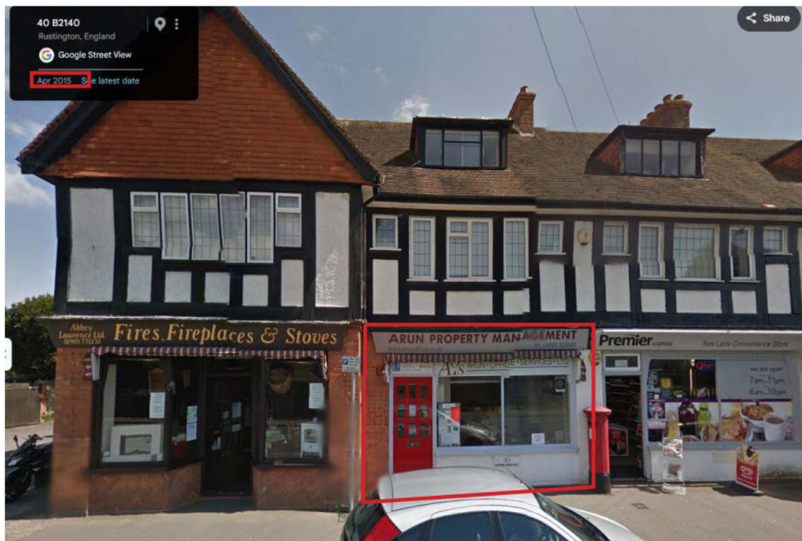
2015: Arun Office Services Ltd / Arun Property Management signage visible at the ground floor premises, 55–57 Sea Lane.
