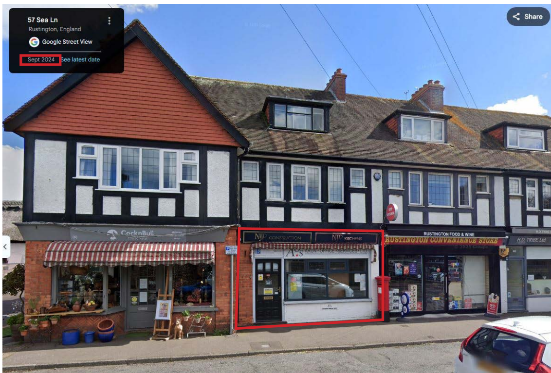
2024: Arun Office Services Ltd / Arun Property Management signage visible at the ground floor premises, 55–57 Sea Lane.
