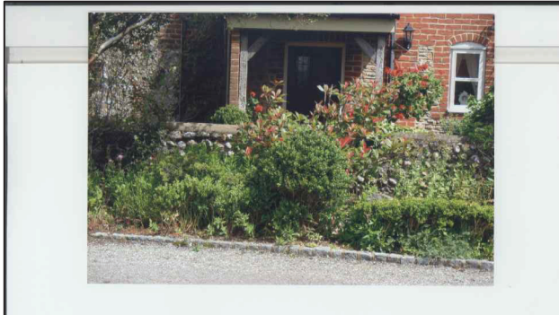
Photo showing existing elevation
