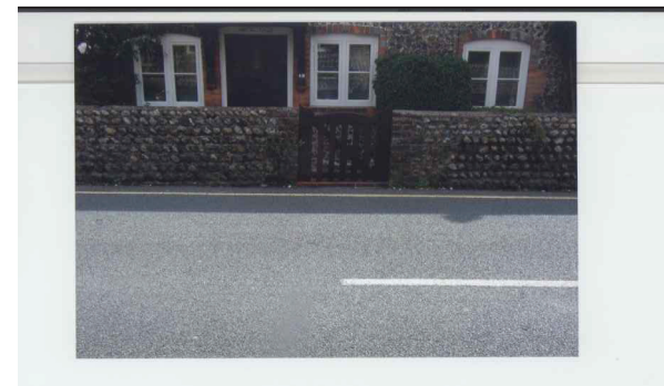
Photo showing existing gate in West elevation
