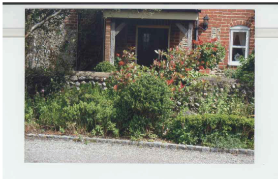
Photo showing existing elevation
