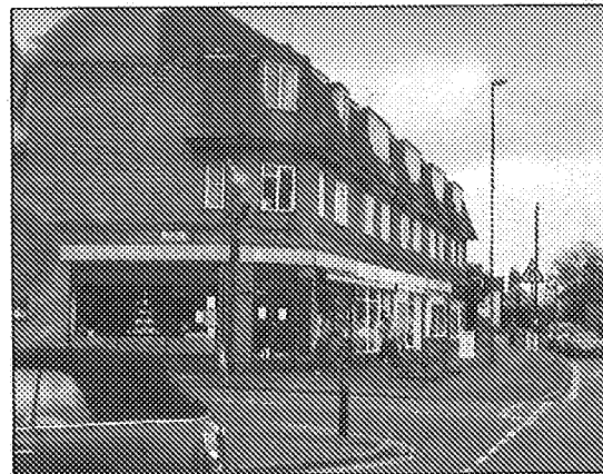
Apartments Sea Lane
