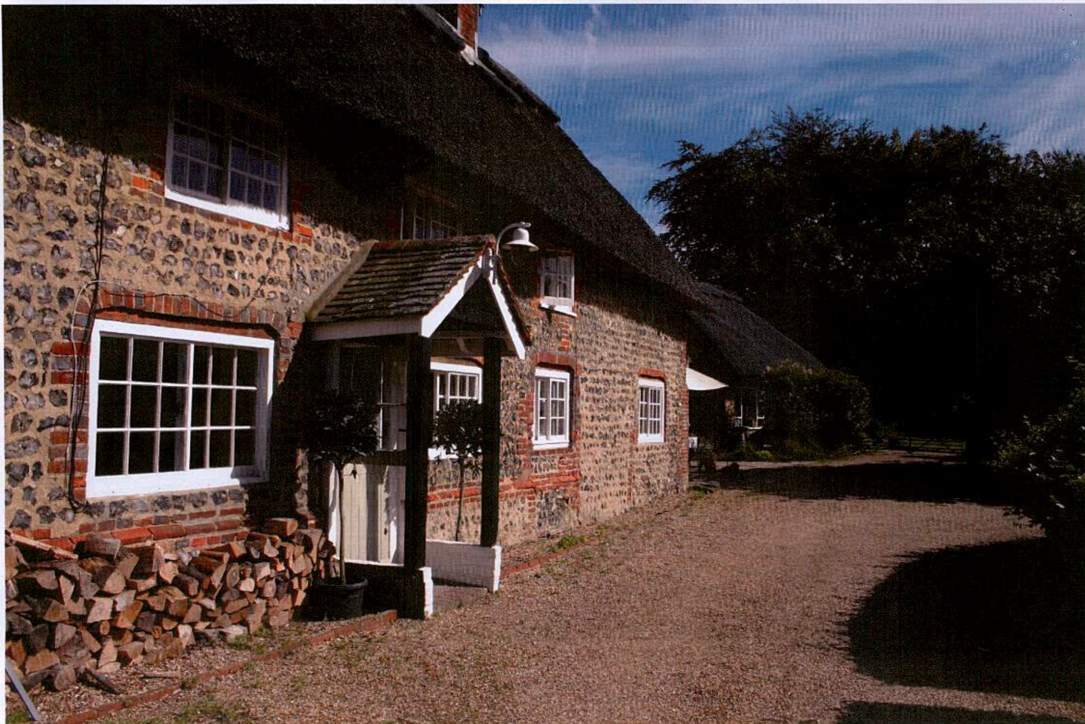
finished work - west elevation
