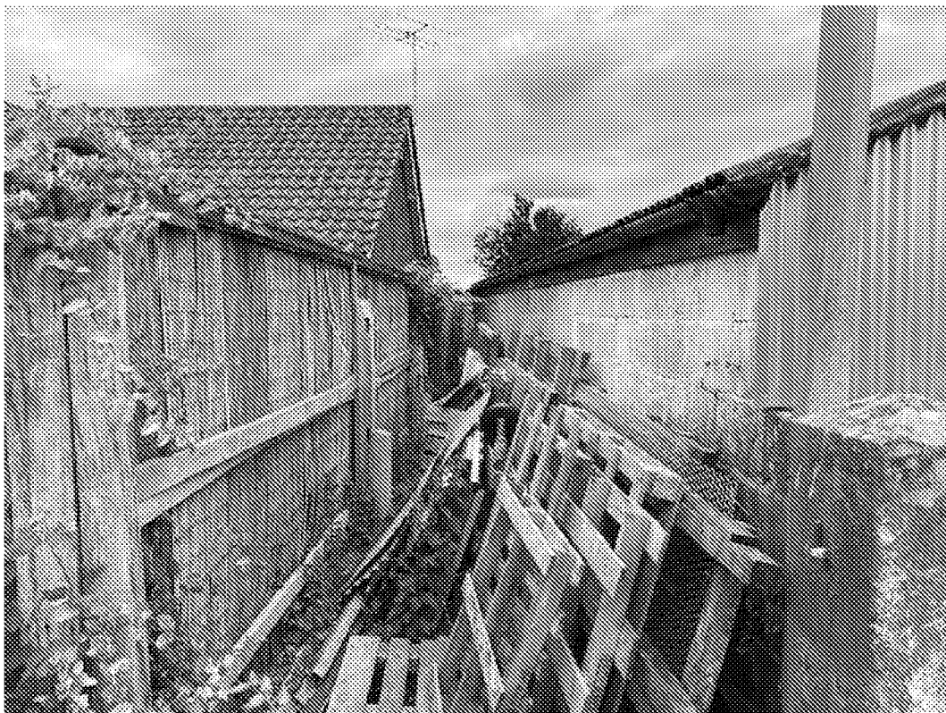
View of northern boundary condition with adjacent bungalow on Fircroft Crescent
