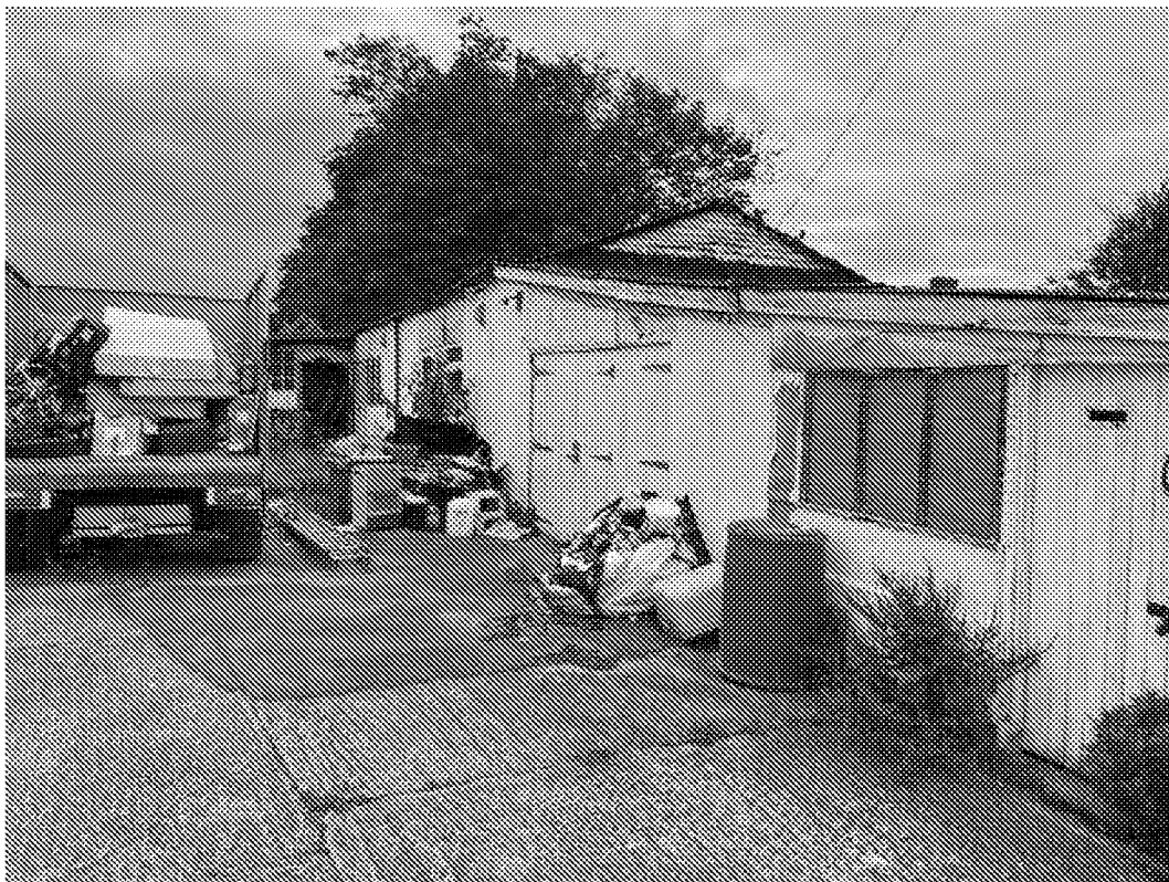
View of existing dilapidated buildings and abandoned vehicles
