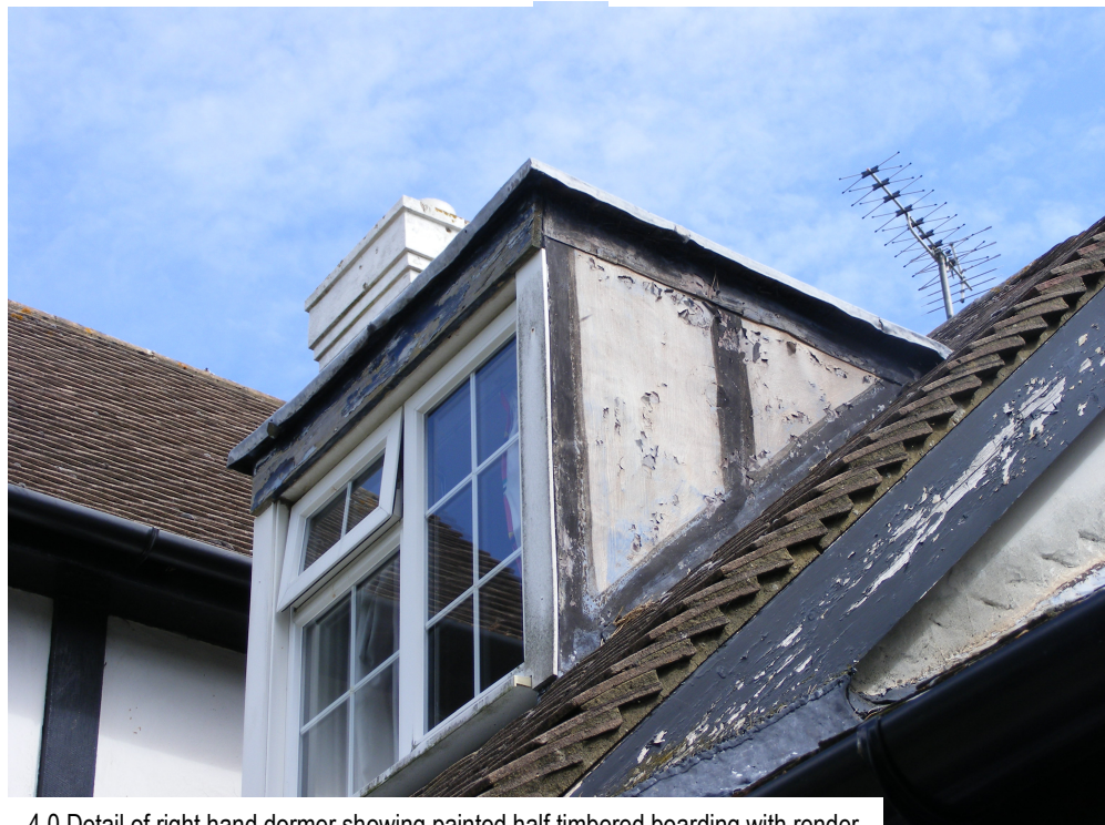
4.0 Detail of right hand dormer showing painted half timbered boarding with render
