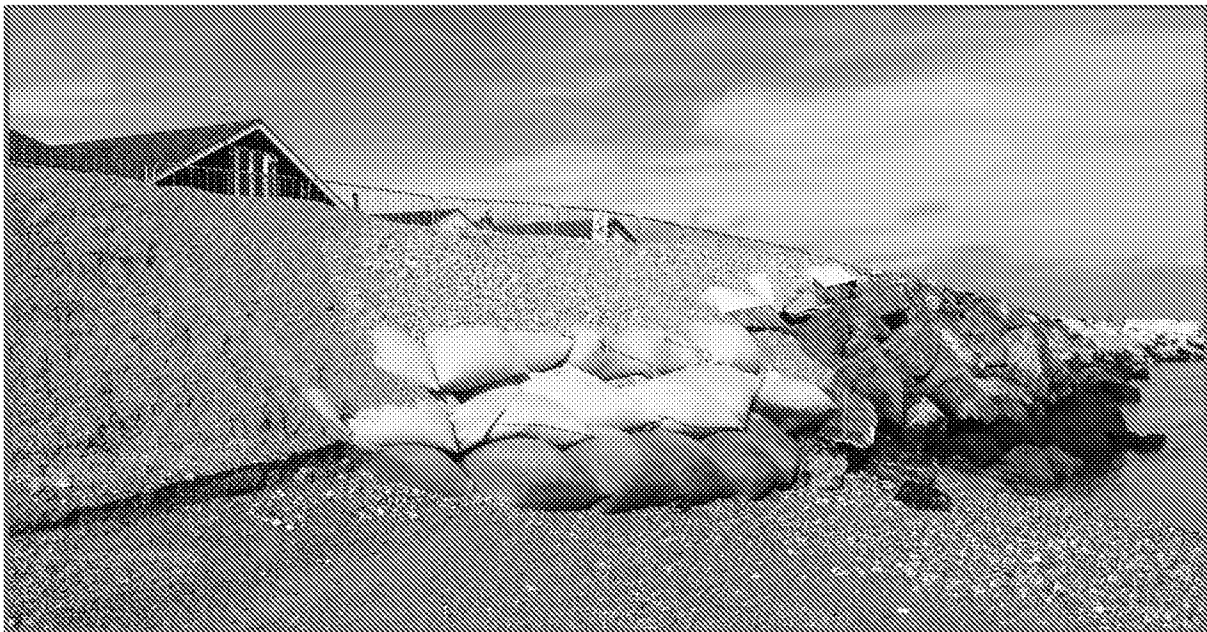
Image 3. Imported rock armouring and exposure of geotextile bags within the inlet channel
