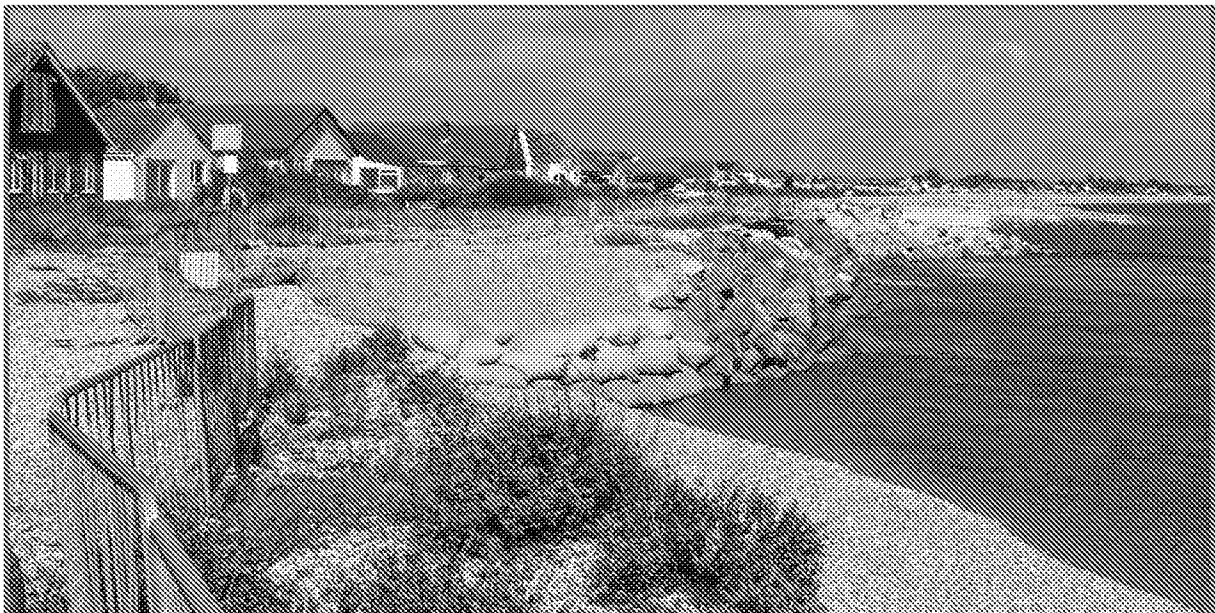
Image 5. Exposure of beach behind rock armour and geotextile bags
