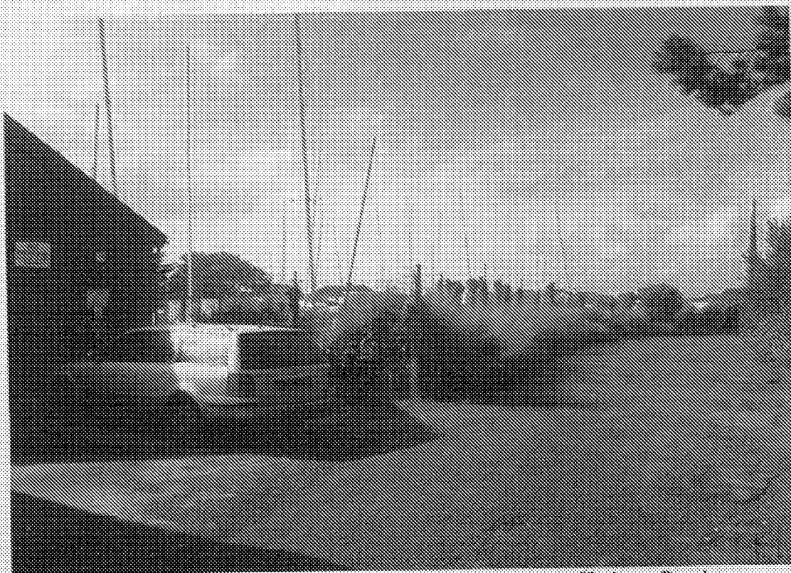
View of the site boundary looking south west along Harbour Road
