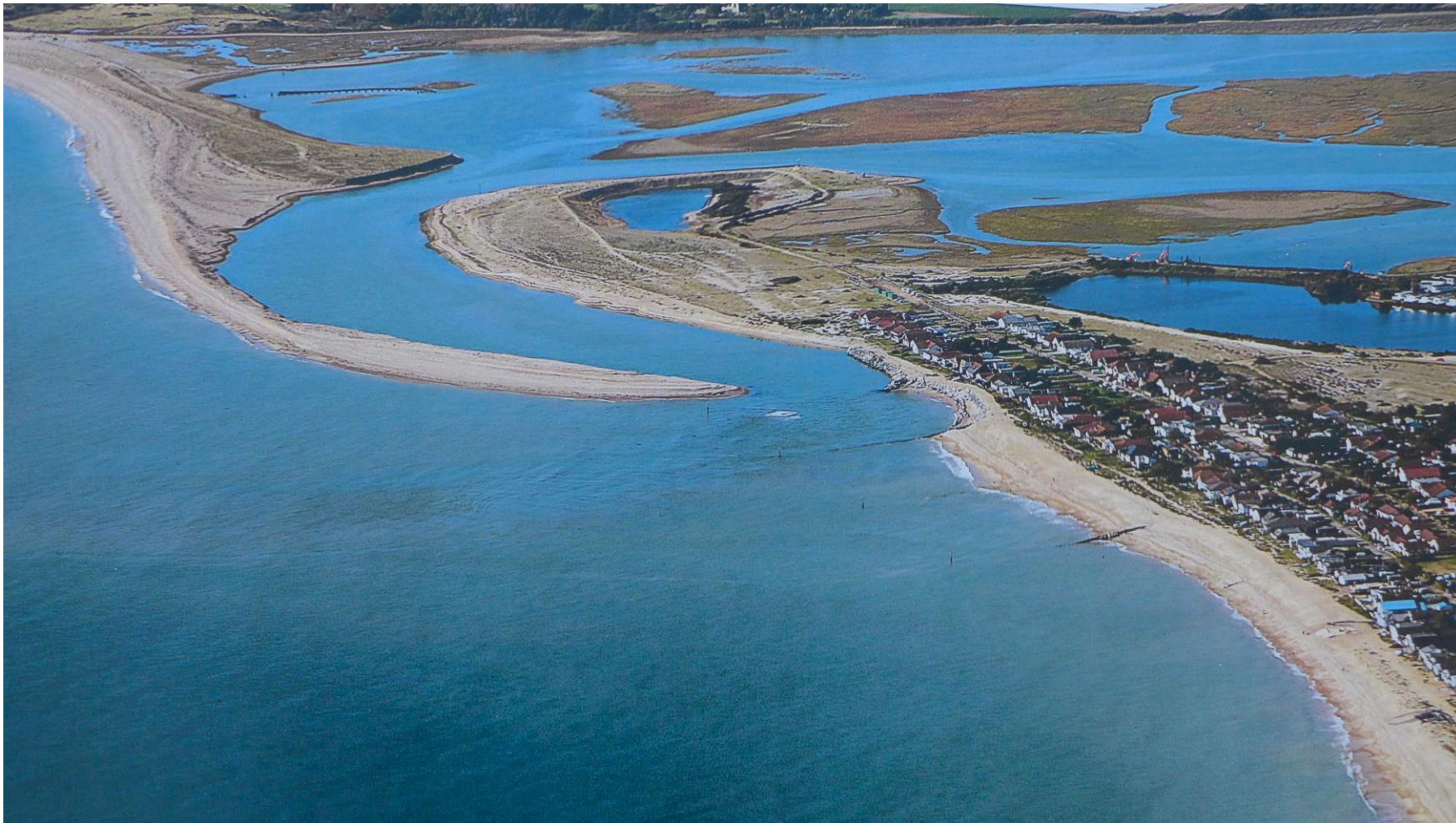
Immediately prior to the breach of CN Spit (25, 26). Early configuration of breach (27 to 35).
