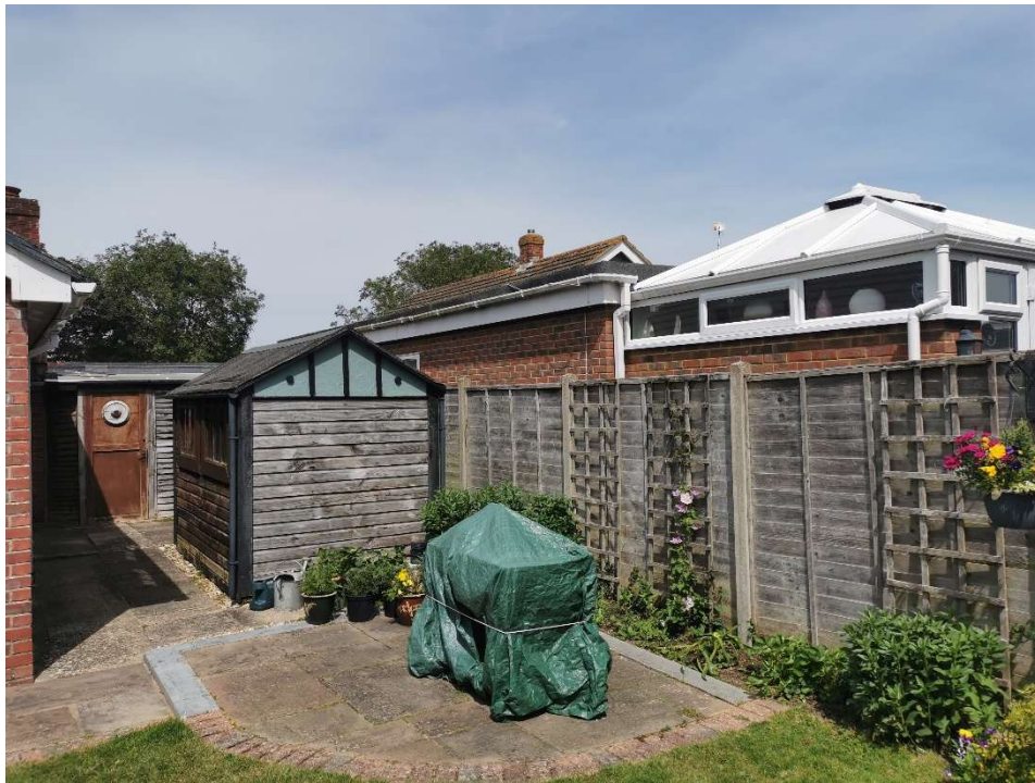
4 – Rear of garage showing neighbouring property
