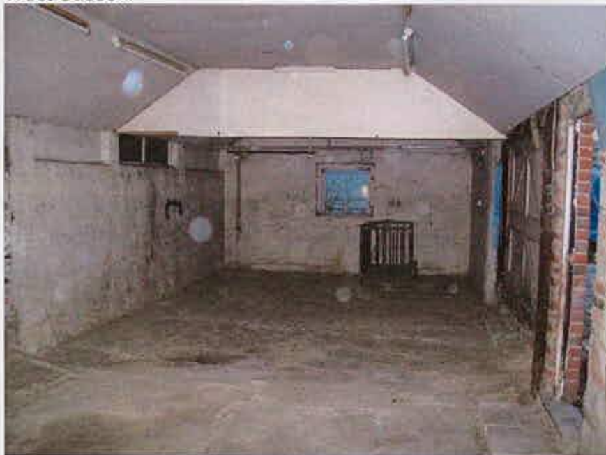
Photograph 2.4: Interior of Building 4, Butterlees Farm, Pagham Road, Lagness, West Sussex.
