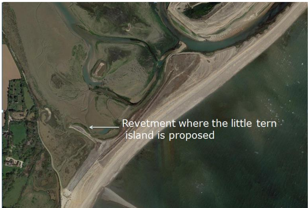
Fig 3: Location of proposed site to create a new little tern nesting spit/islet on the Church Norton side of the harbour. This is the site of the 1910 breach and includes old concrete revetments from the previously installed training wall overlying a bed of shingle.
