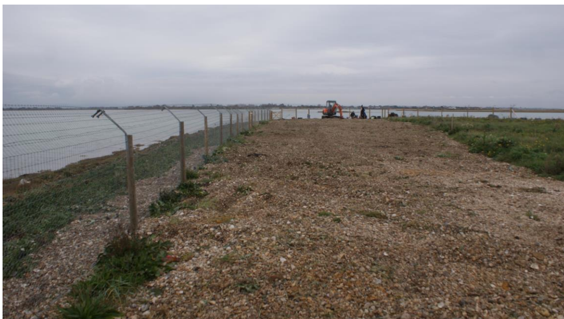
Fig 6. – Predator fence and shingle nesting habitat just after installation (Tern Island Pagham Harbour - April 2018
