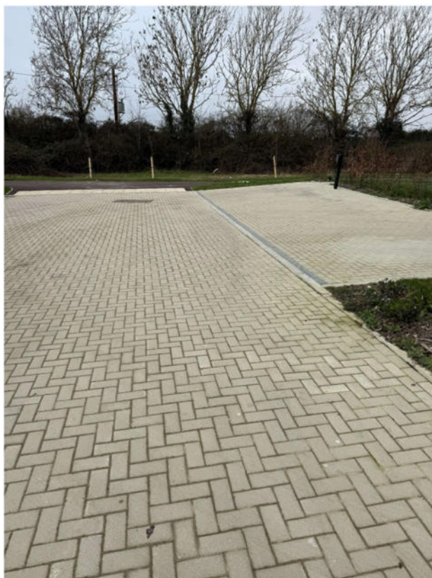
Figure 7 – Road gullies opposite plot 31
