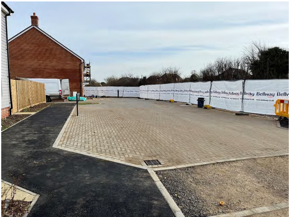
Figure 3 - Road gully in 298/300 access road
