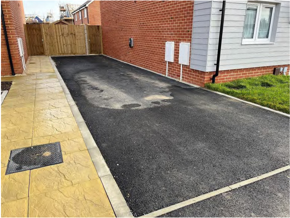
Figure 5 - Plot 296 drive with on-plot drainage installed in line with design drawings
