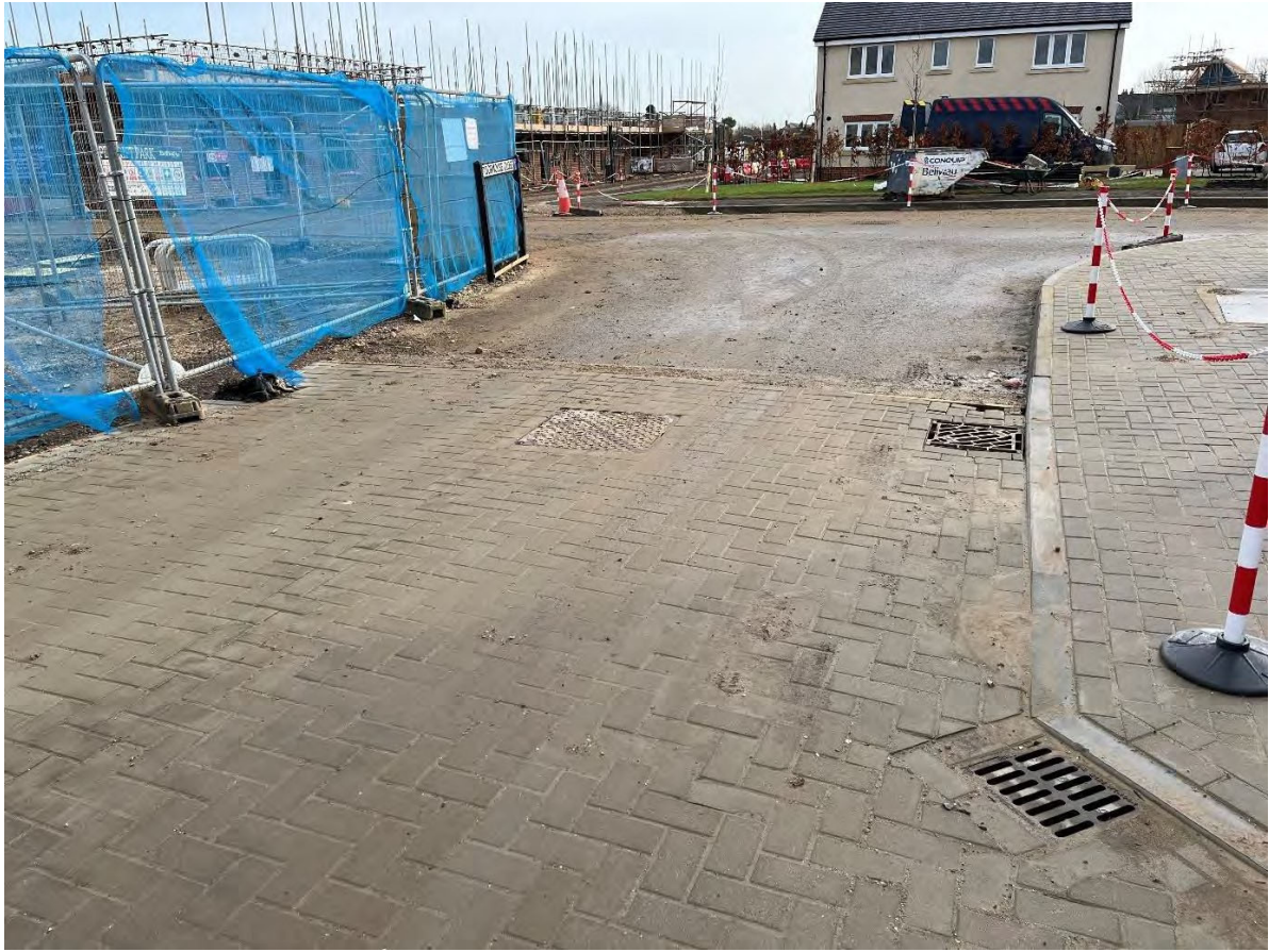
Figure 1 - Road gullies by junction adjacent to plot 9
