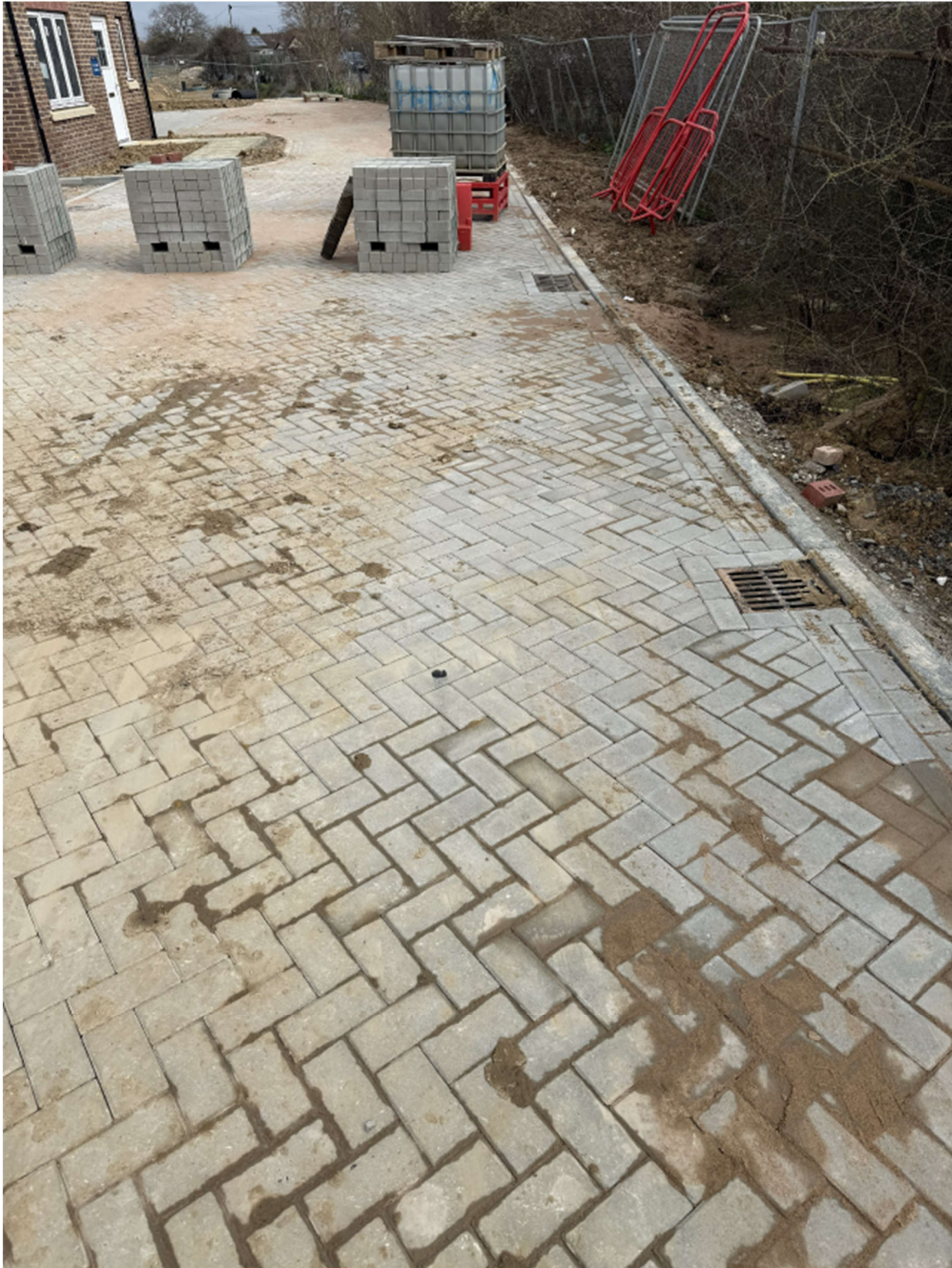
Figure 11 – Road gullies in access road outside Plot 268
