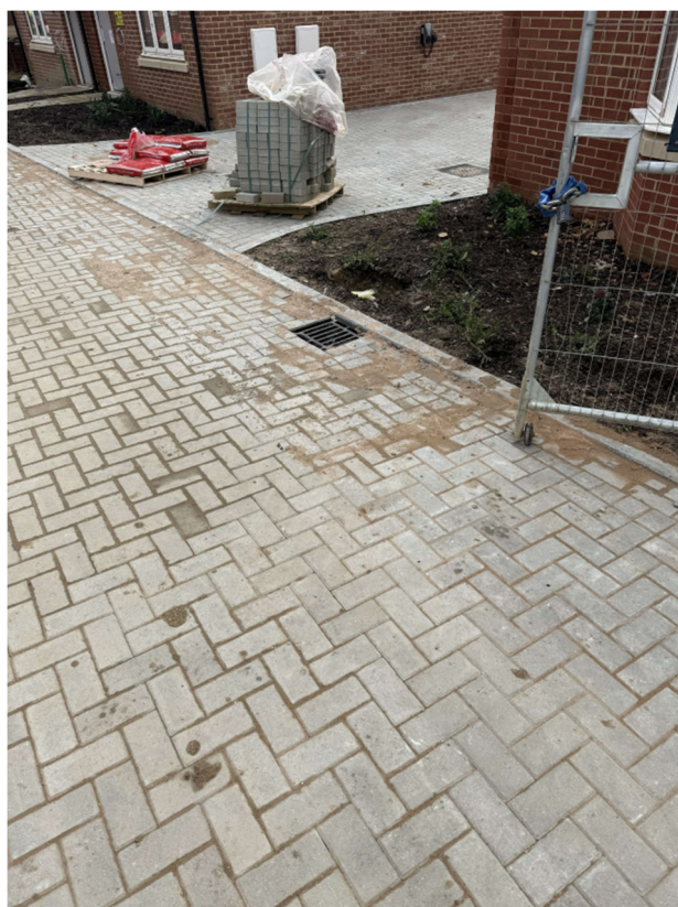
Figure 10 – Road gullies in access outside Plot 265
