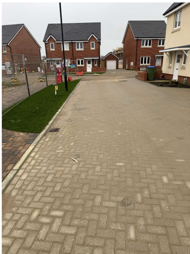
Figure 9 – Road gullies in access road to Plots 40 – 43
