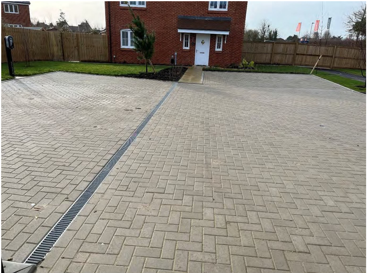
Figure 2 - Drainage channel within plot 12/13 parking area
