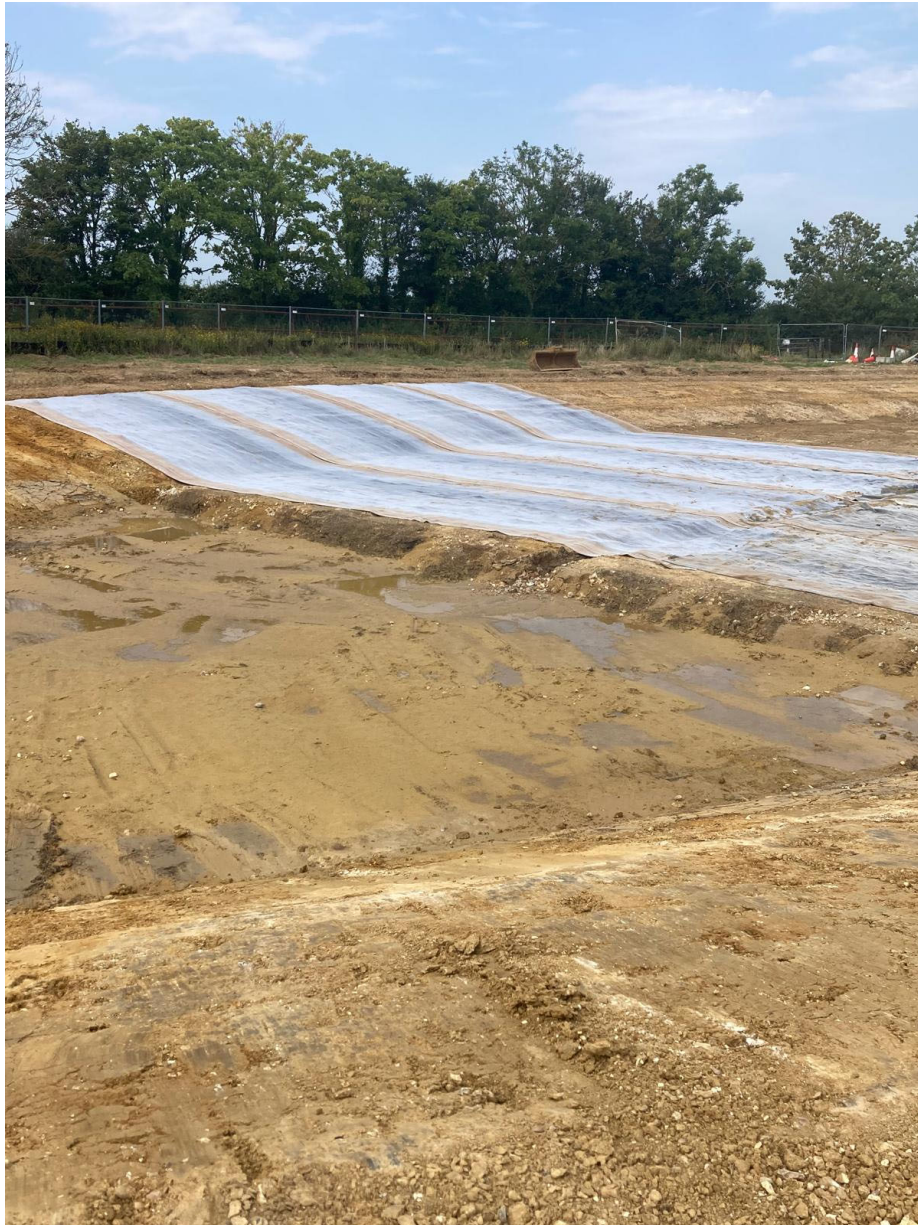
BASIN 3 construction photos
