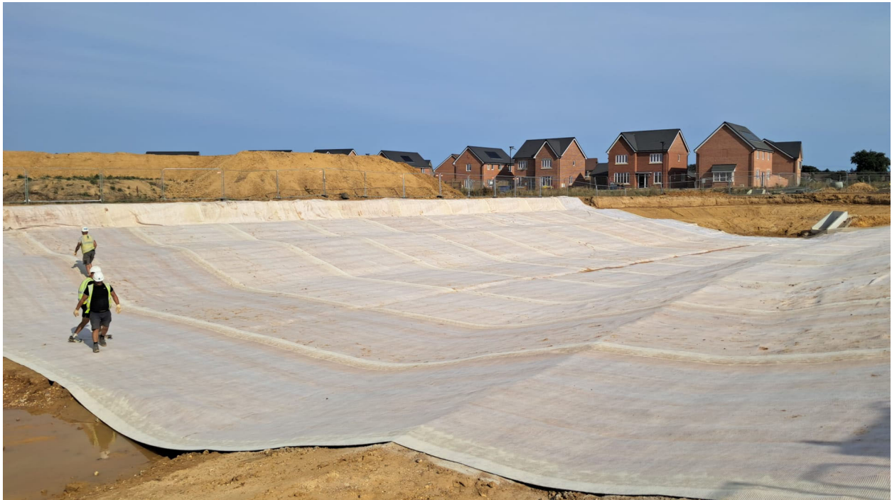
BASIN 2 construction photos
