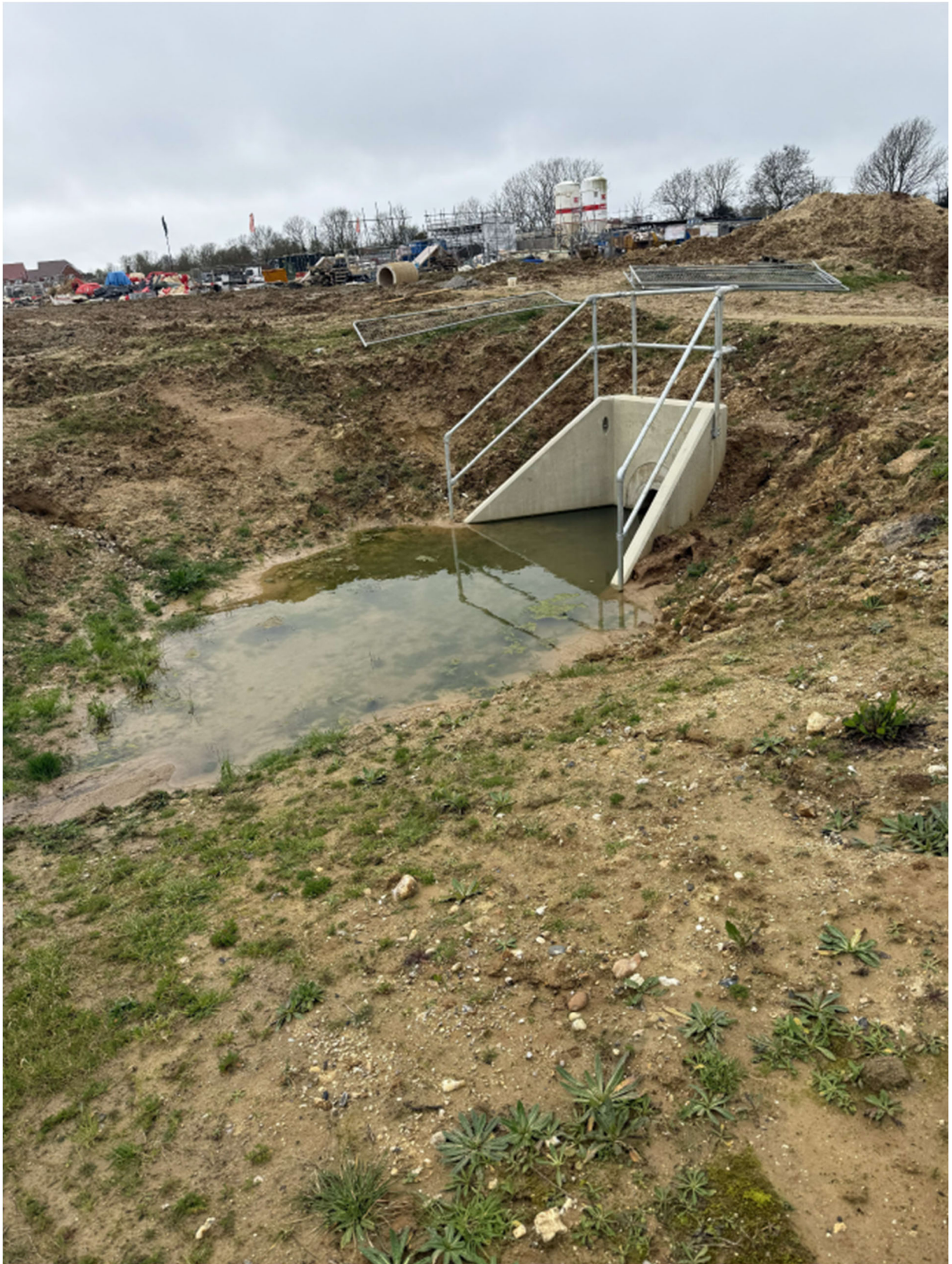
Figure 17 – View of Culvert 4 towards outlet Headwall 07
