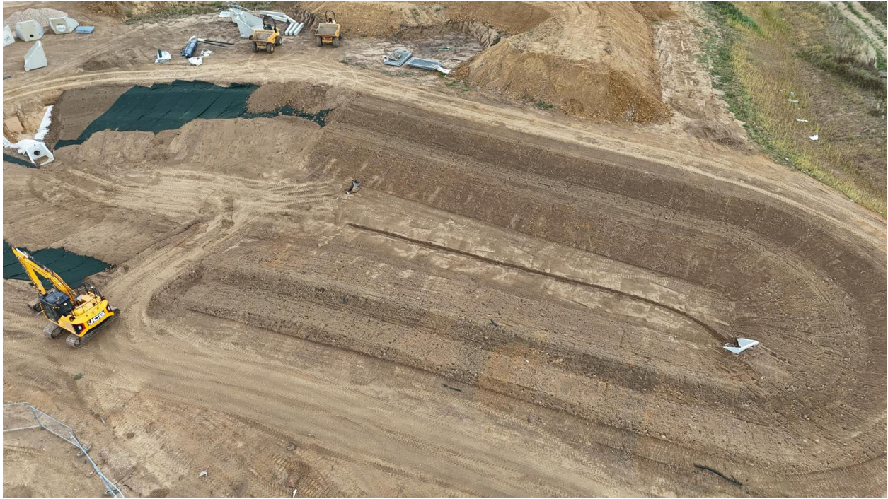
BASIN 2 construction photos
