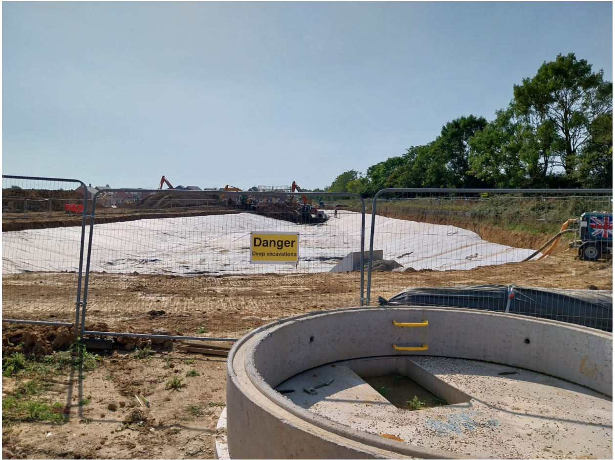
BASIN 1A construction photos
