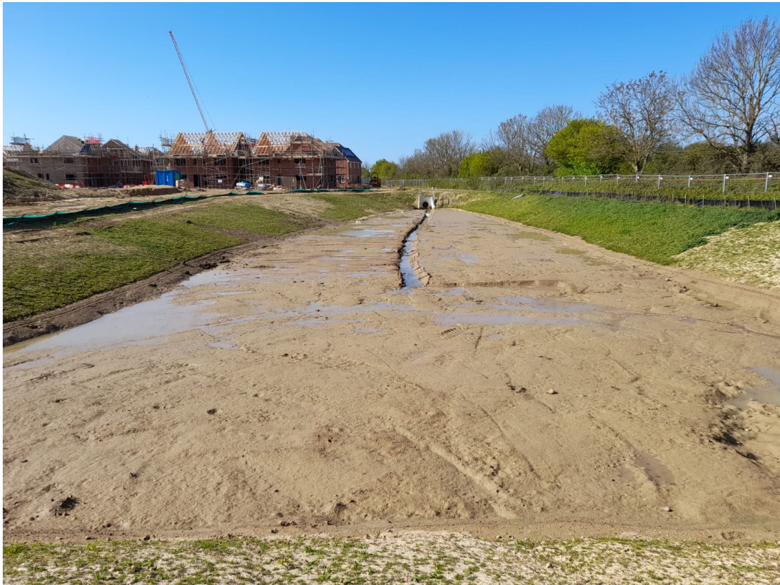
BASIN 1B construction photos
