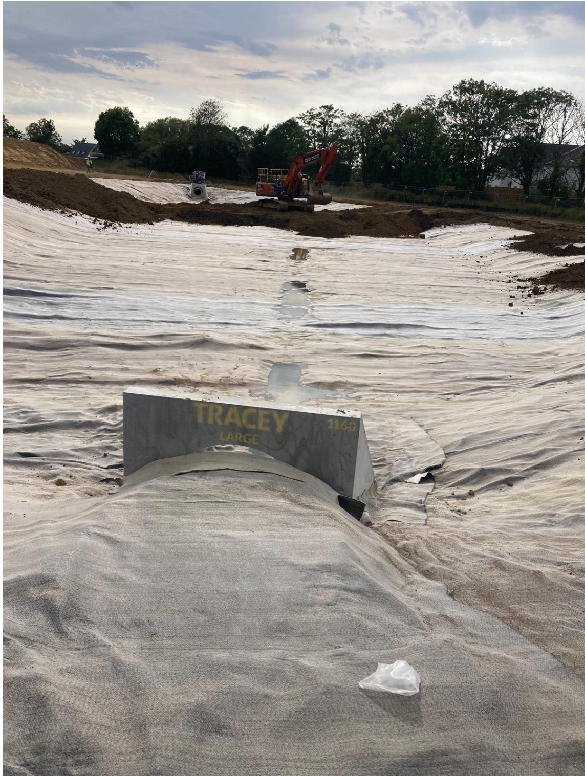
BASIN 3 construction photos
