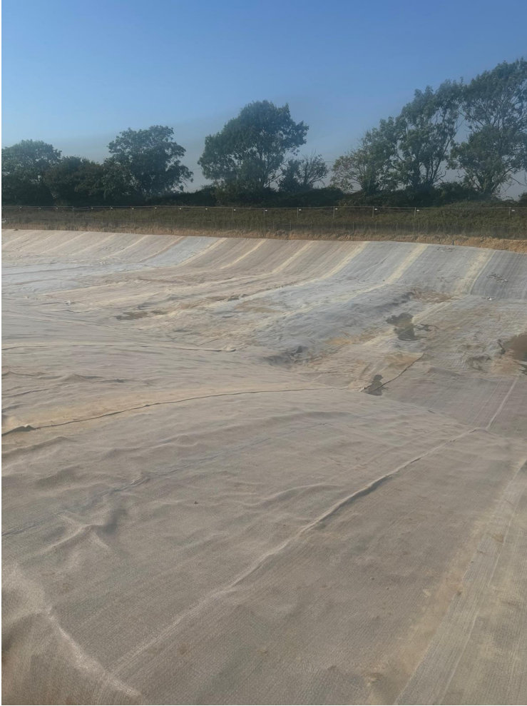
BASIN 1A construction photos
