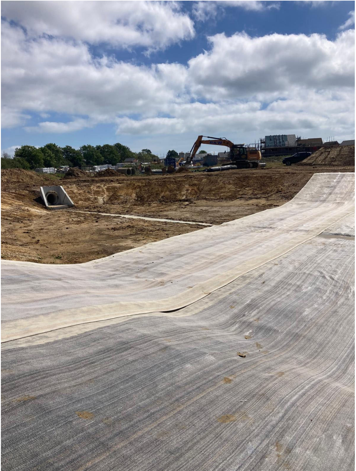
BASIN 3 construction photos
