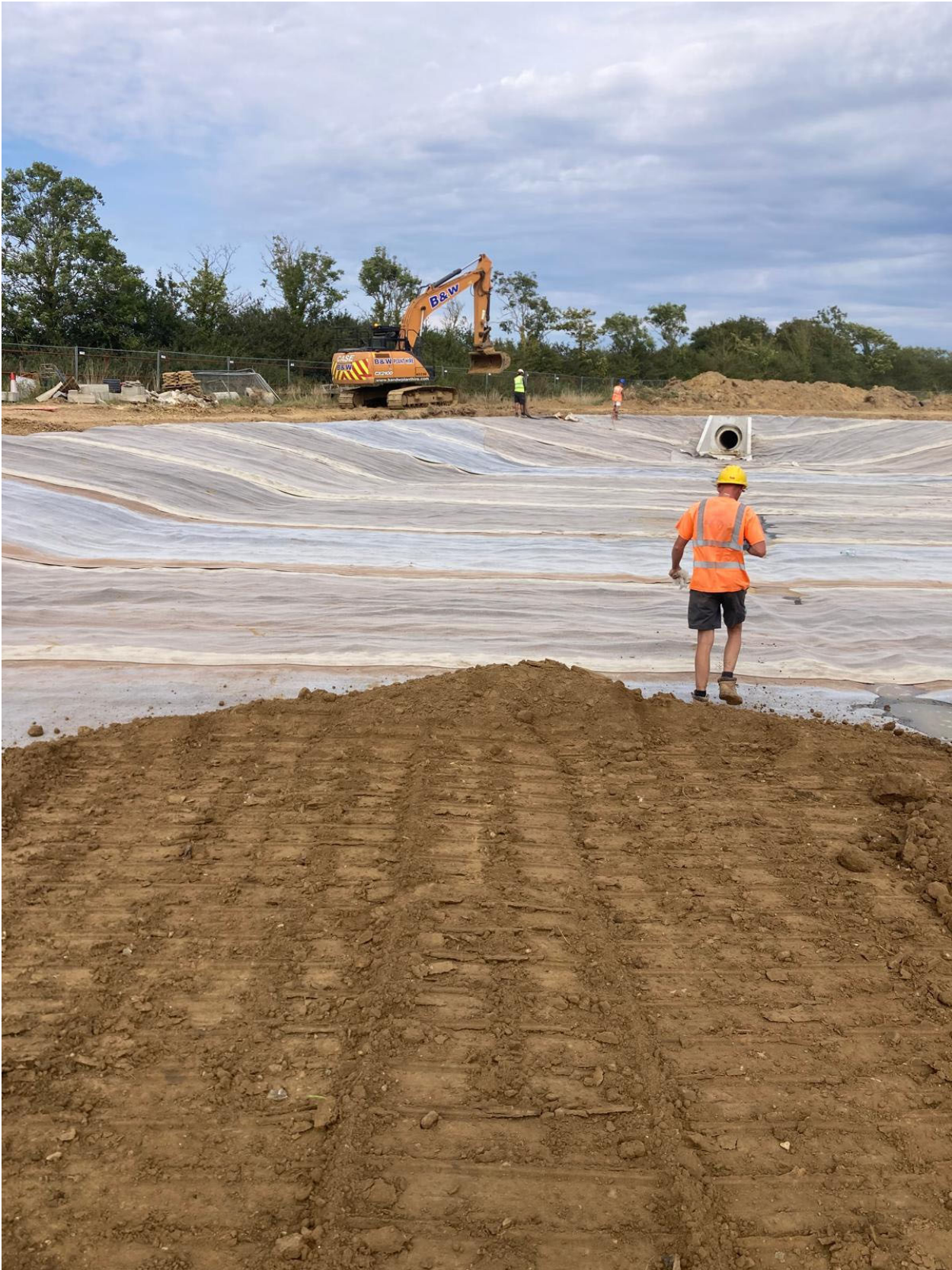
BASIN 3 construction photos
