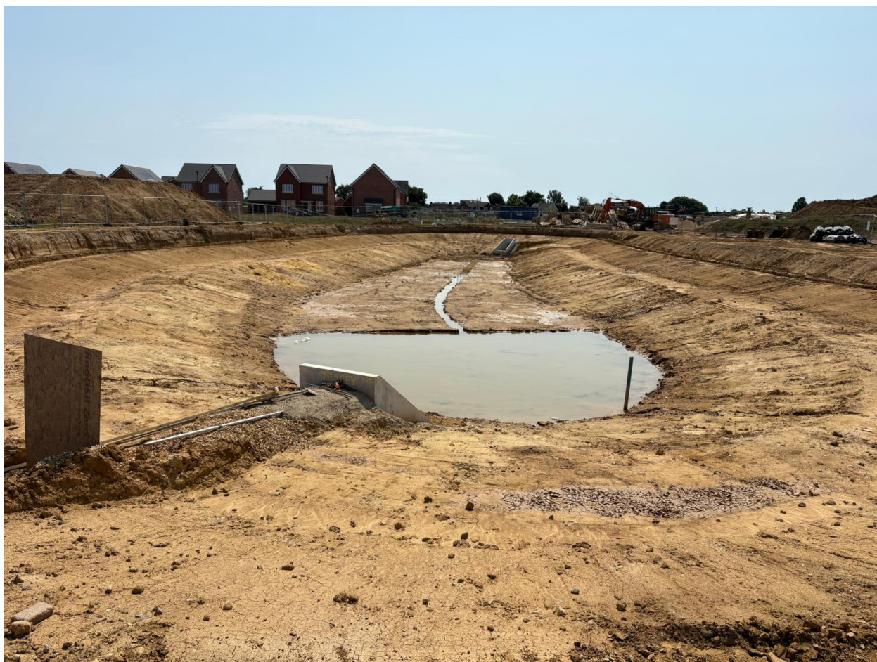
Figure 13 - View of Basin 2 during construction towards H15
