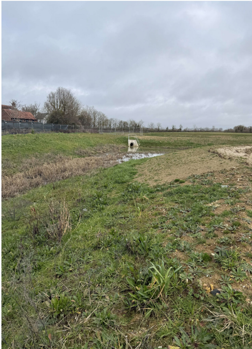
Figure 9 – View of Basin 1B towards outlet Headwall 13
