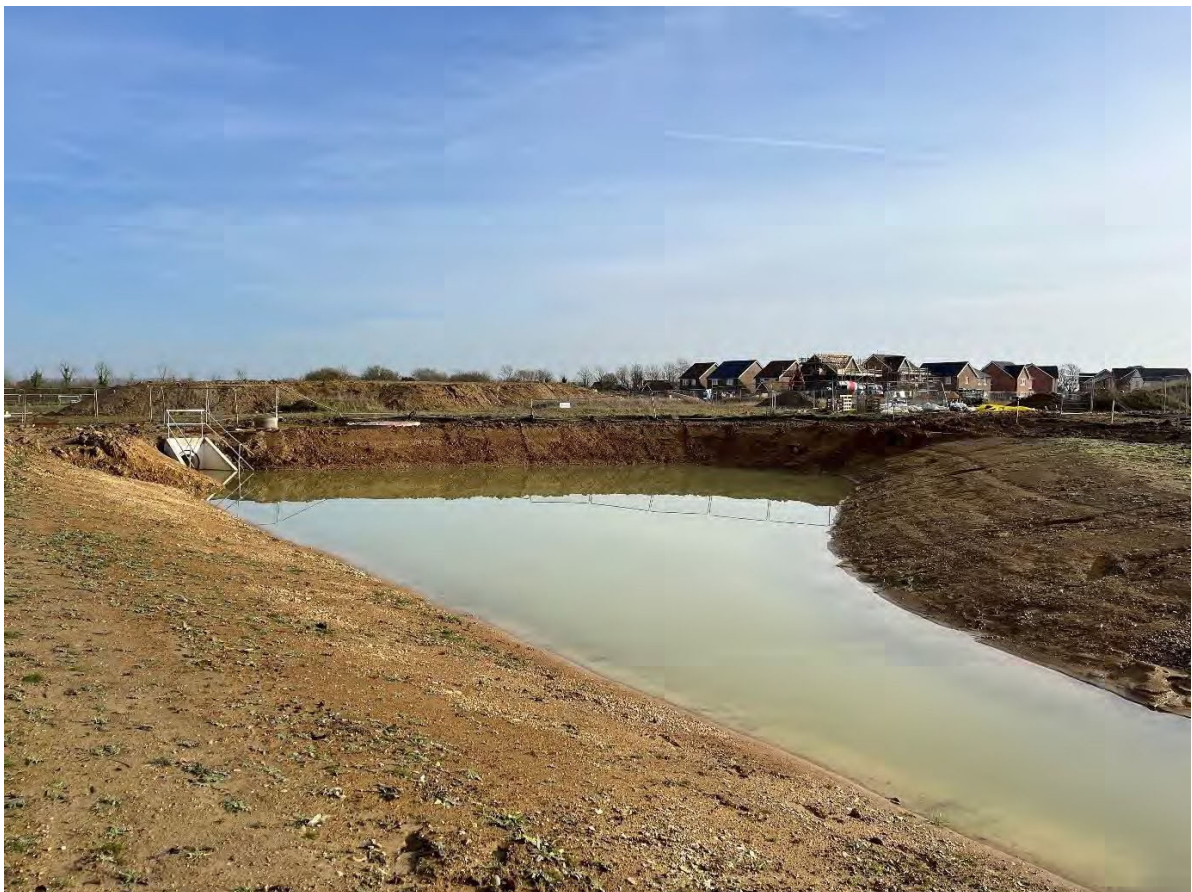
Figure 6 - View of Basin 1B
