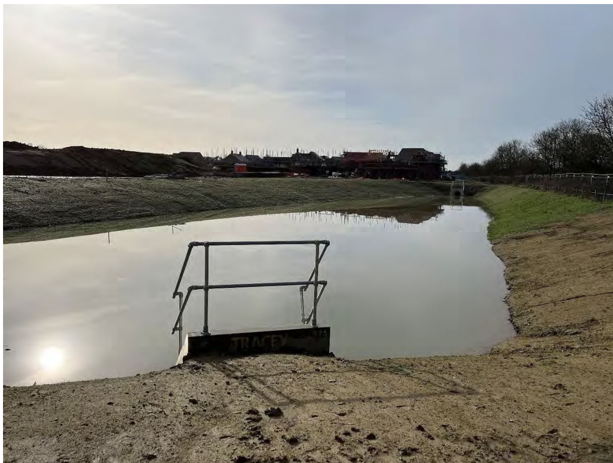
Figure 1. View of Basin 1A from outlet headwall HW11 towards HW09
