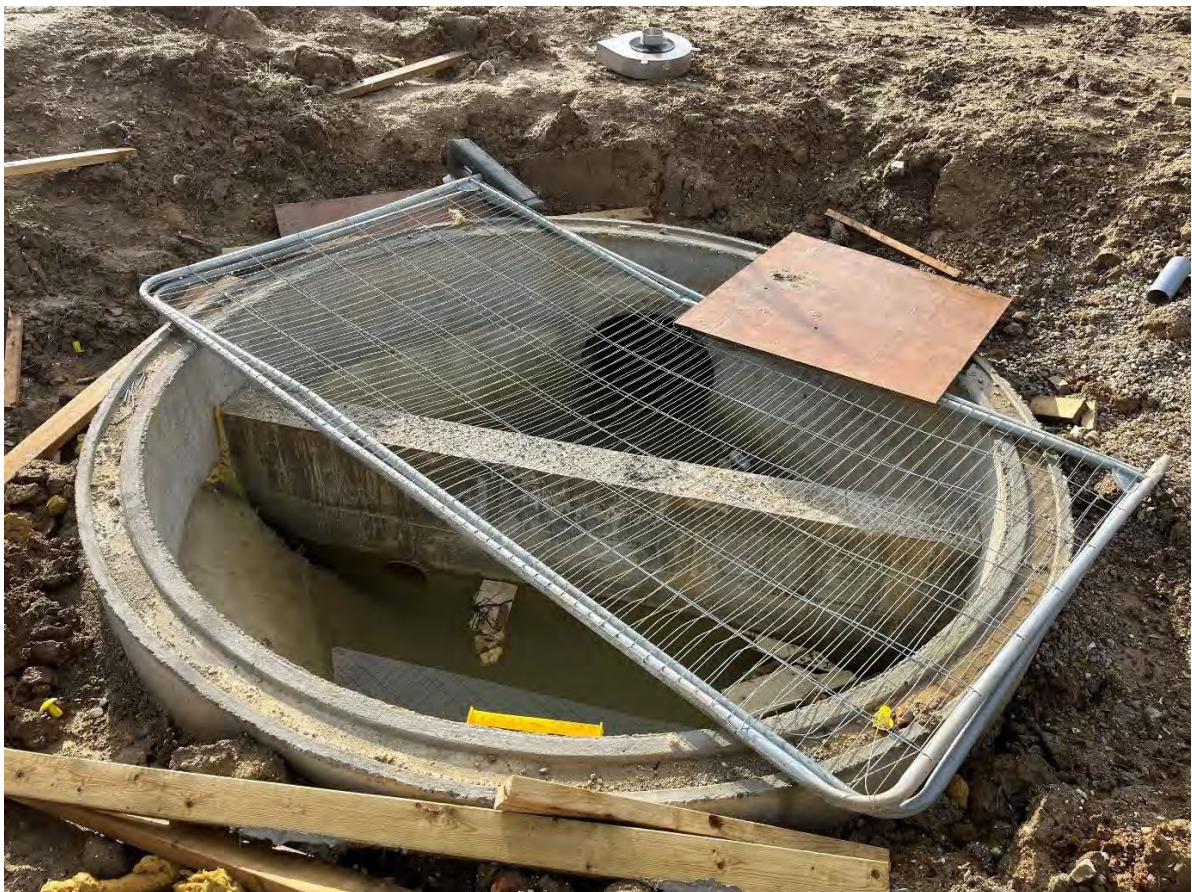
Figure 8 - Flow control manhole S54 still under construction
