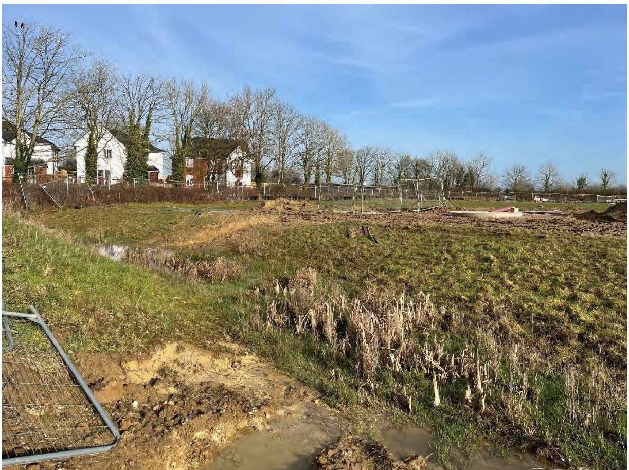
Figure 12 - View of new watercourse from outfall looking west
