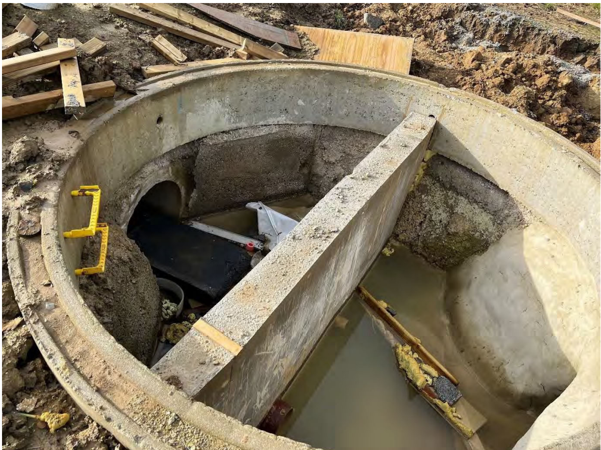
Figure 4 - Flow control manhole S43 still under construction
