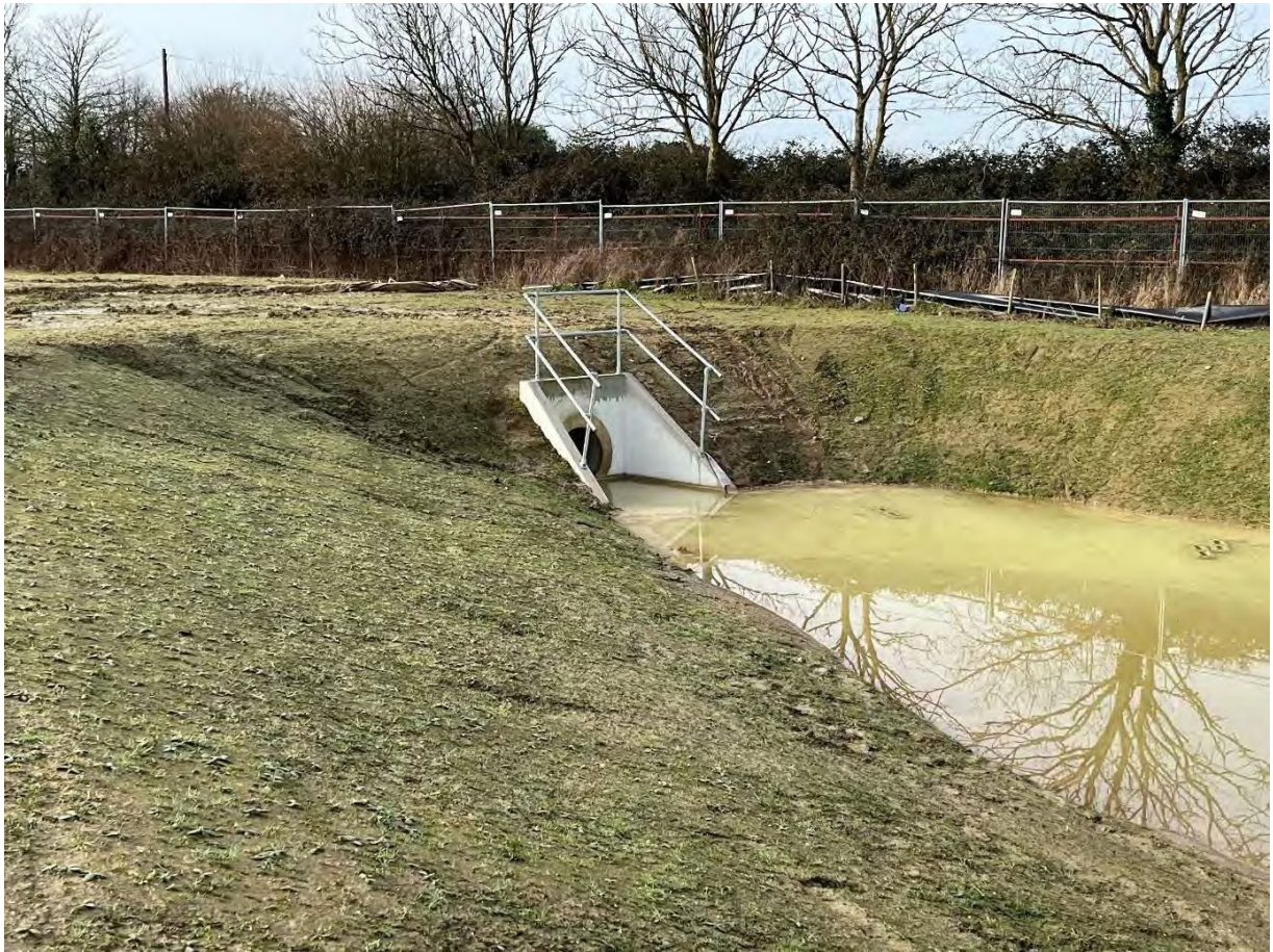
Figure 3 - Basin 1A inlet headwall HW09
