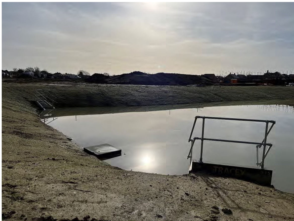
Figure 2 - View of Basin 1A from outlet headwall HW11 towards HW10
