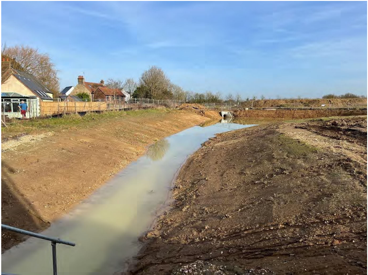
Figure 5 - View of Basin 1B from inlet headwall HW12
