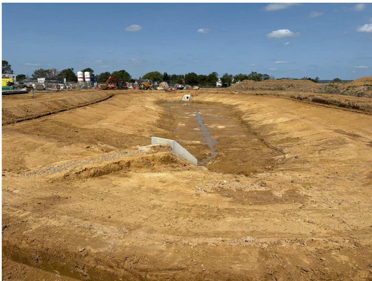
Figure 14 - View of Basin 2 during construction towards H16
