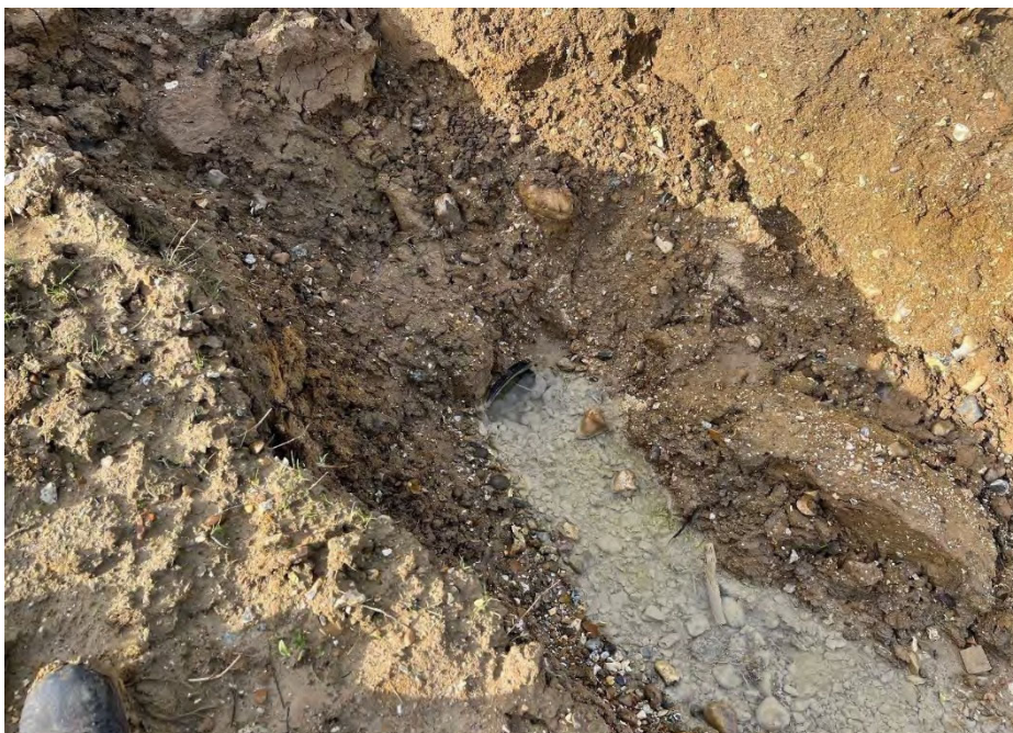
Figure 10 - Outfall pipe into new watercourse with headwall HW14 still to be installed
