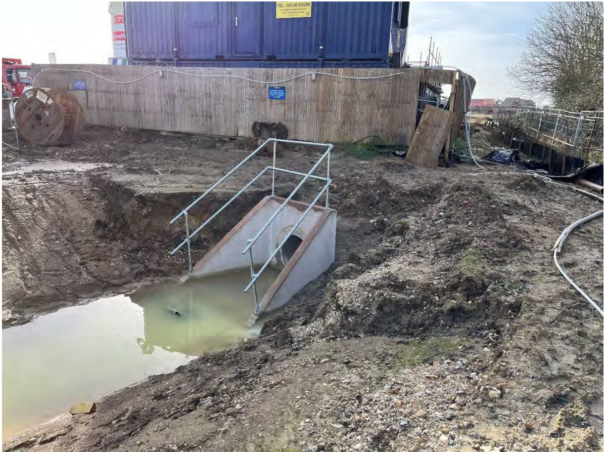
Figure 7 – Basin 1B inlet headwall HW12
