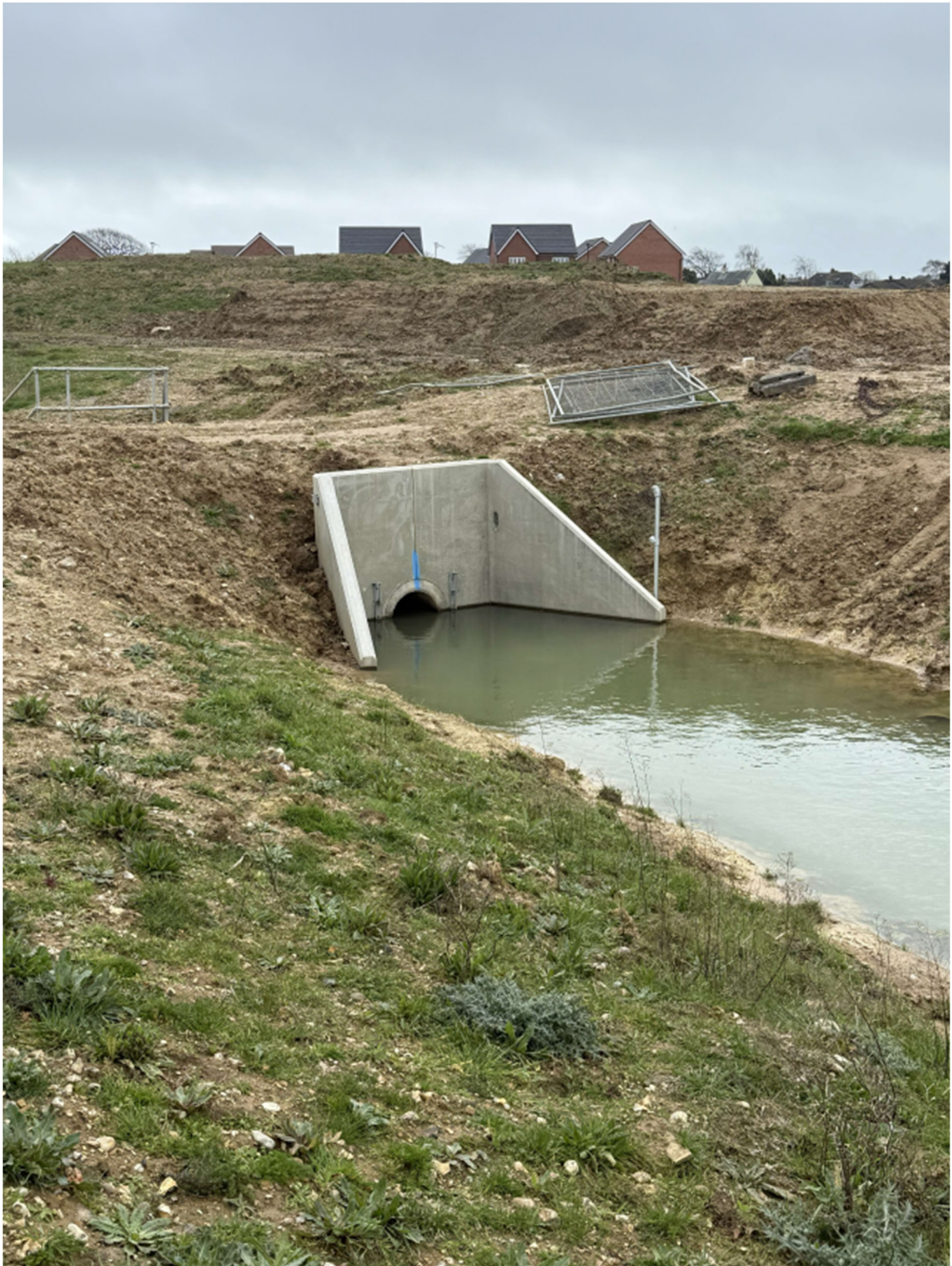
Figure 16 – View of Culvert 4 towards outlet Headwall 08
