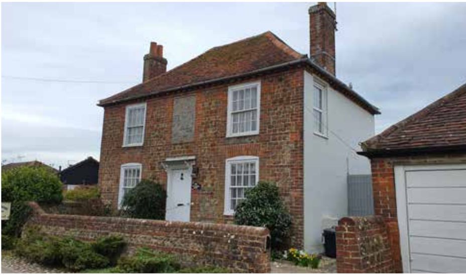
Top: Detached bungalows with buff brick and landscape-oriented windows Bottom: Georgian cottage with portrait-oriented windows
