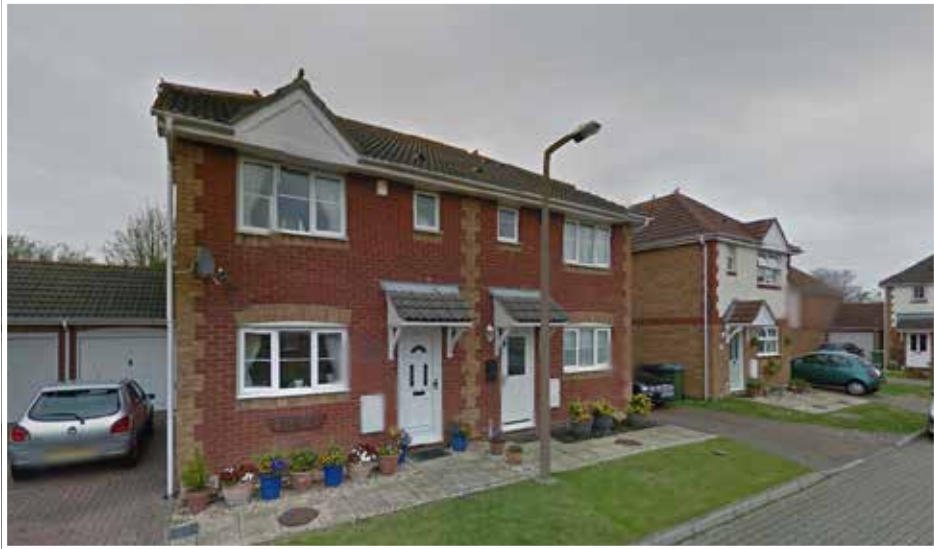
Top: Semi-detached house with hipped roof, stone cills and stone lintels Bottom: Semi-detached house with mono-pitched canopy and contrast brick quoining, cills and lintels
