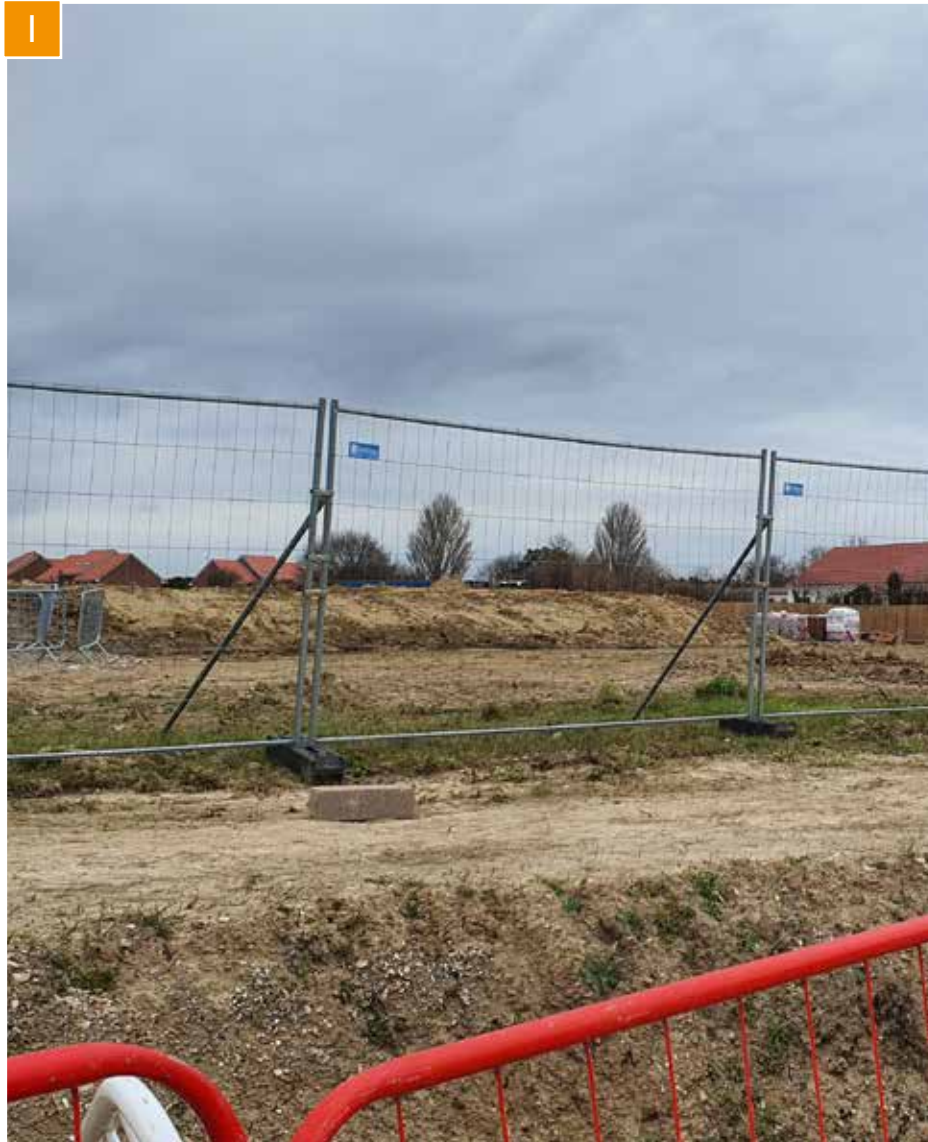
View of adjacent building site north of Summer Lane
