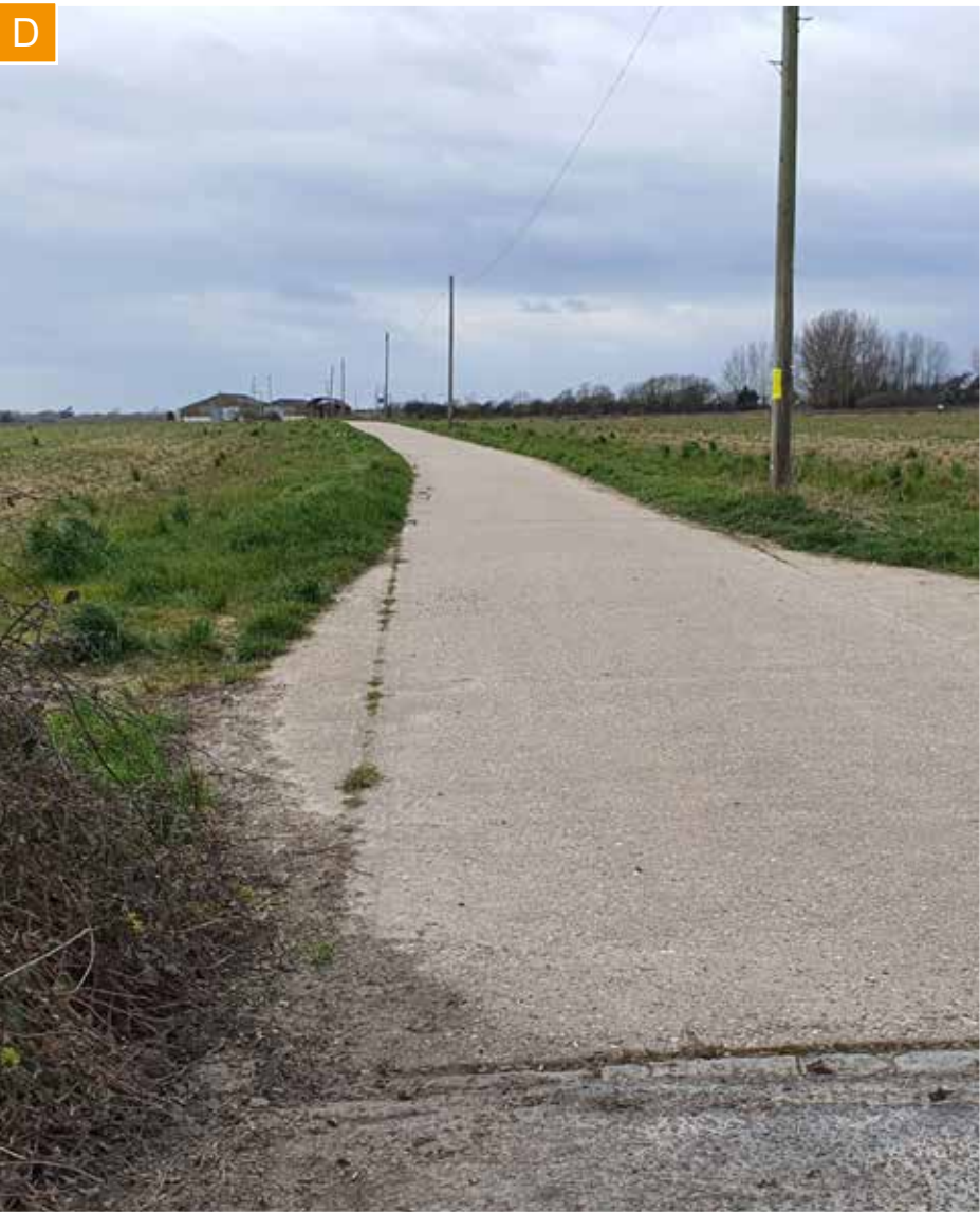
View down the public right of way that separates the southern parcel from the community hub parcel
