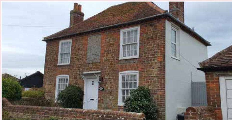
Precedent: Georgian house on Barton Close
