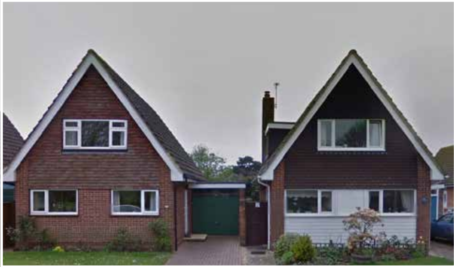
Top: Semi detached house with pale brick and contrast banding Bottom: Detached one-and-a-half storey homes with tile hanging
