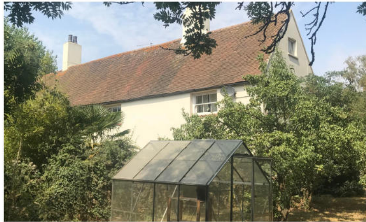
Figure 4 Photograph of Sefter Farmhouse
