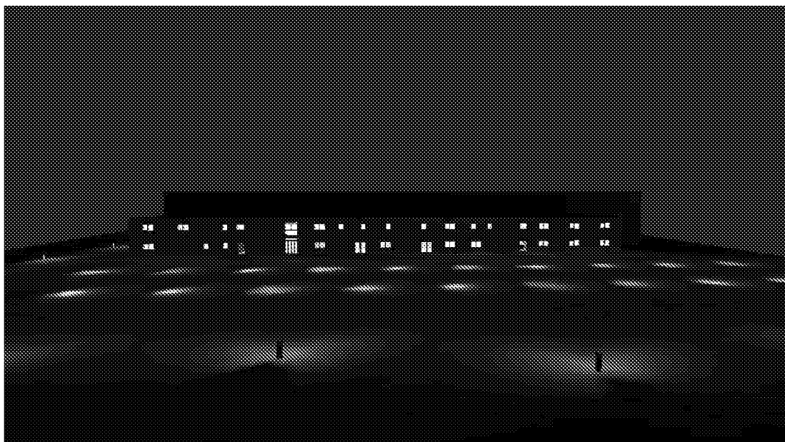
View of the offices looking across the car park
