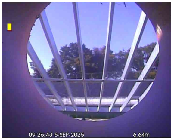
RESEVOIRX_bdc79af6-eead-4f66-b5d9-a2f8449b14dd_2025 0910_083717_304.jpg, 00:00:54, 6.64 m Finish node, outfall, reference: RESEVOIR
