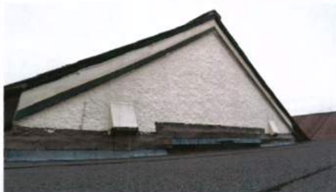
RANGE OF ROOF REPAIRS
