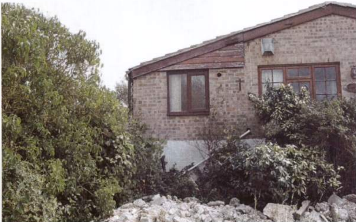
Photograph No. 1 - North-Eastern Elevation of Main Building on Site. Negligible Nesting opportunities for Swallow or Starling respectively. Ventilation hole in centre of Photograph is closed.
