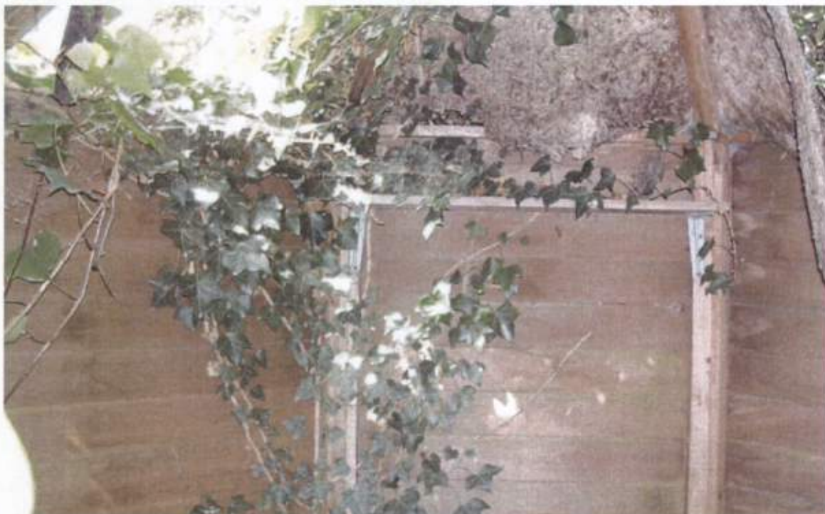
Photograph No. 12 - Potential Nesting Space for Swallows at juncture of Wall and Roof in Octagonal Shed found at Northern End of Site.
