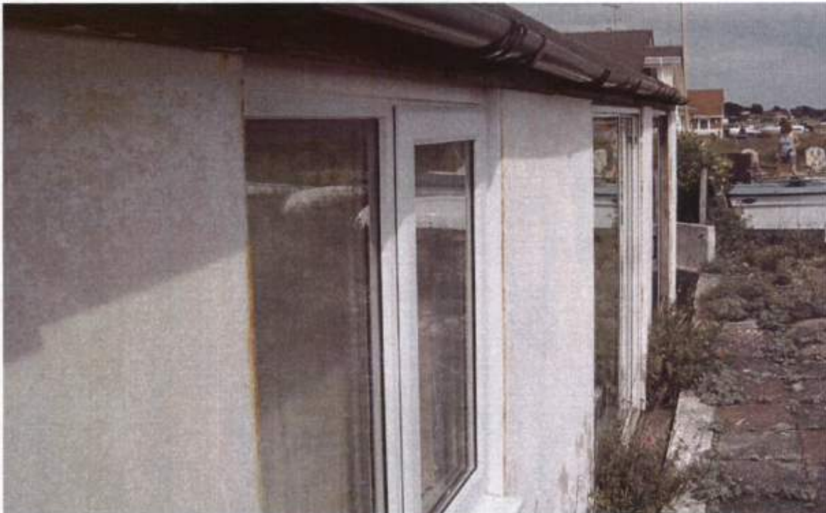
Photograph No. 5 - South-Eastern Elevation of Main Building on Site. Negligible Nesting opportunities for Swallow or Starling respectively.
