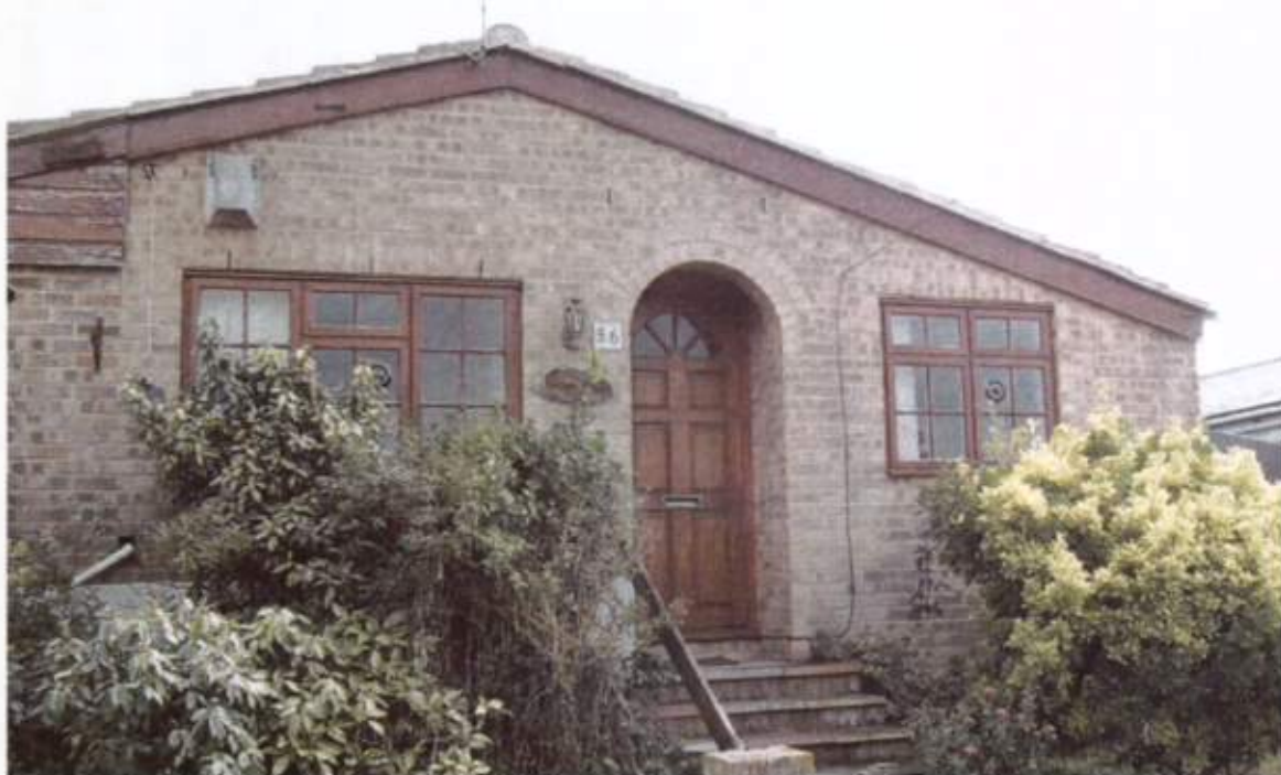
Photograph No. 2 - North-Eastern Elevation of Main Building on Site. Negligible Nesting opportunities for Swallow or Starling respectively.
