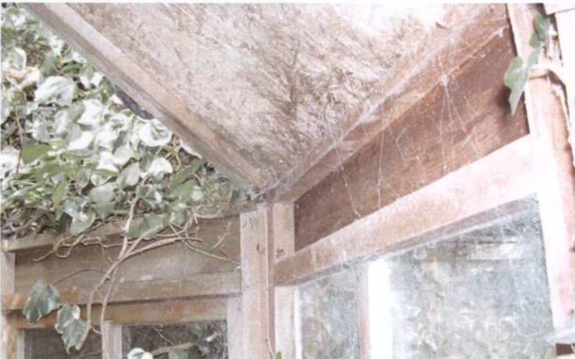
Photograph No. 14 - Potential Nesting Space for Swallows at juncture of Wall and Roof in Octagonal Shed found at Northern End of Site.
