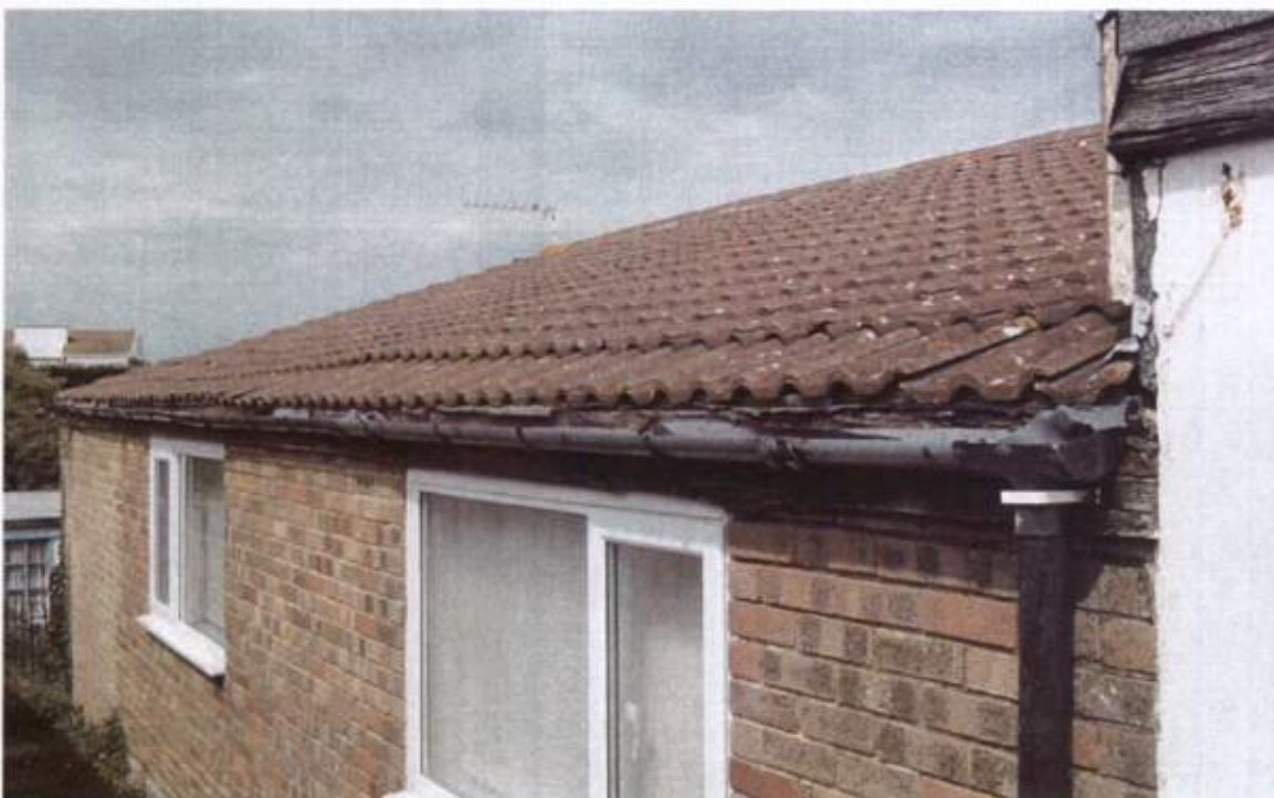
Photograph No. 4 - South-Western Elevation and Roof of Main Building on Site. Negligible Nesting opportunities for Swallow or Starling respectively.
