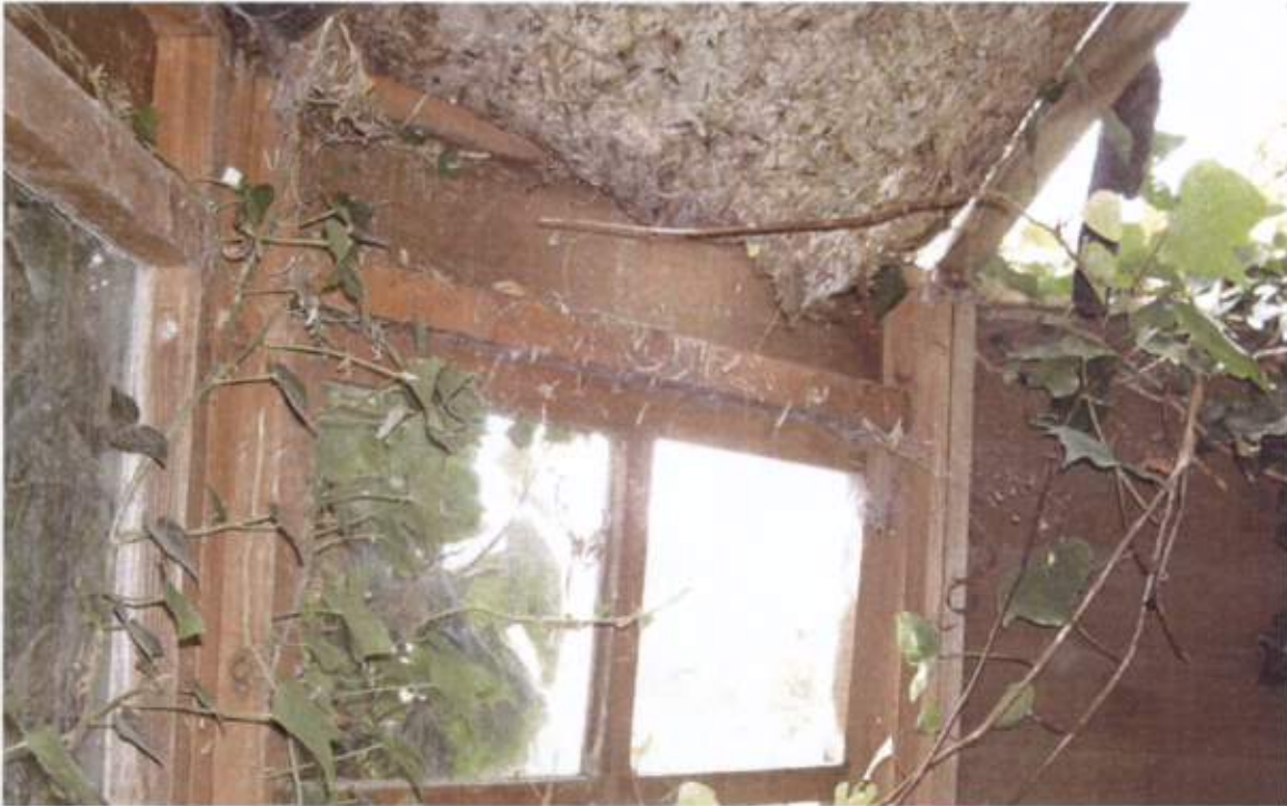
Photograph No. 13 - Potential Nesting Space for Swallows at juncture of Wall and Roof in Octagonal Shed found at Northern End of Site.
