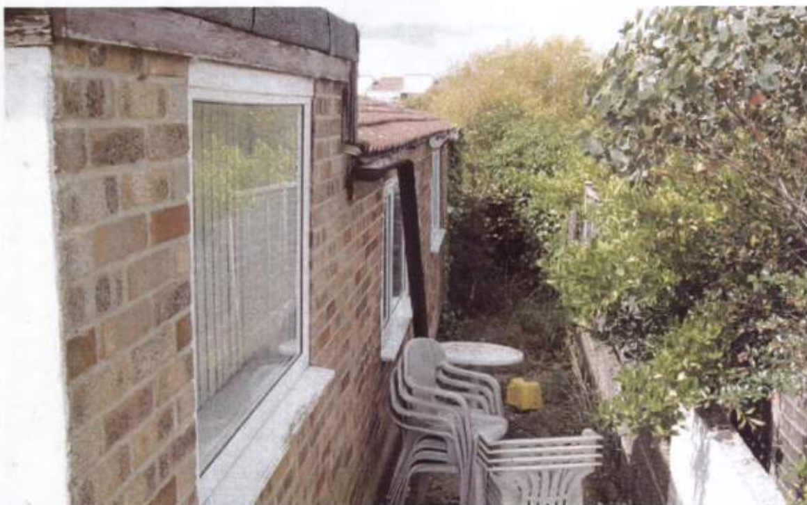
Photograph No. 7 - North-Eastern Elevation of Main Building on Site. Negligible Nesting opportunities for Swallow or Starling respectively.
