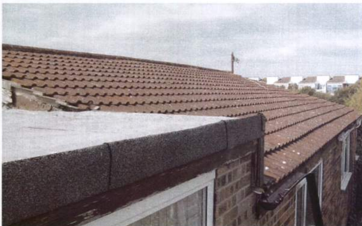
Photograph No. 8 - North-Eastern Roof of Main Building on Site. Negligible Nesting opportunities for Swallow or Starling respectively.
