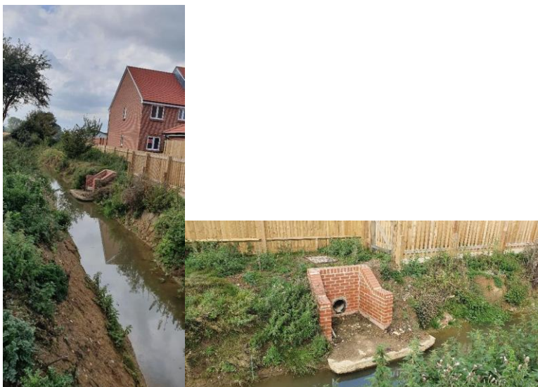
Photo 6&7 -looking west and north towards Crayfern Development
