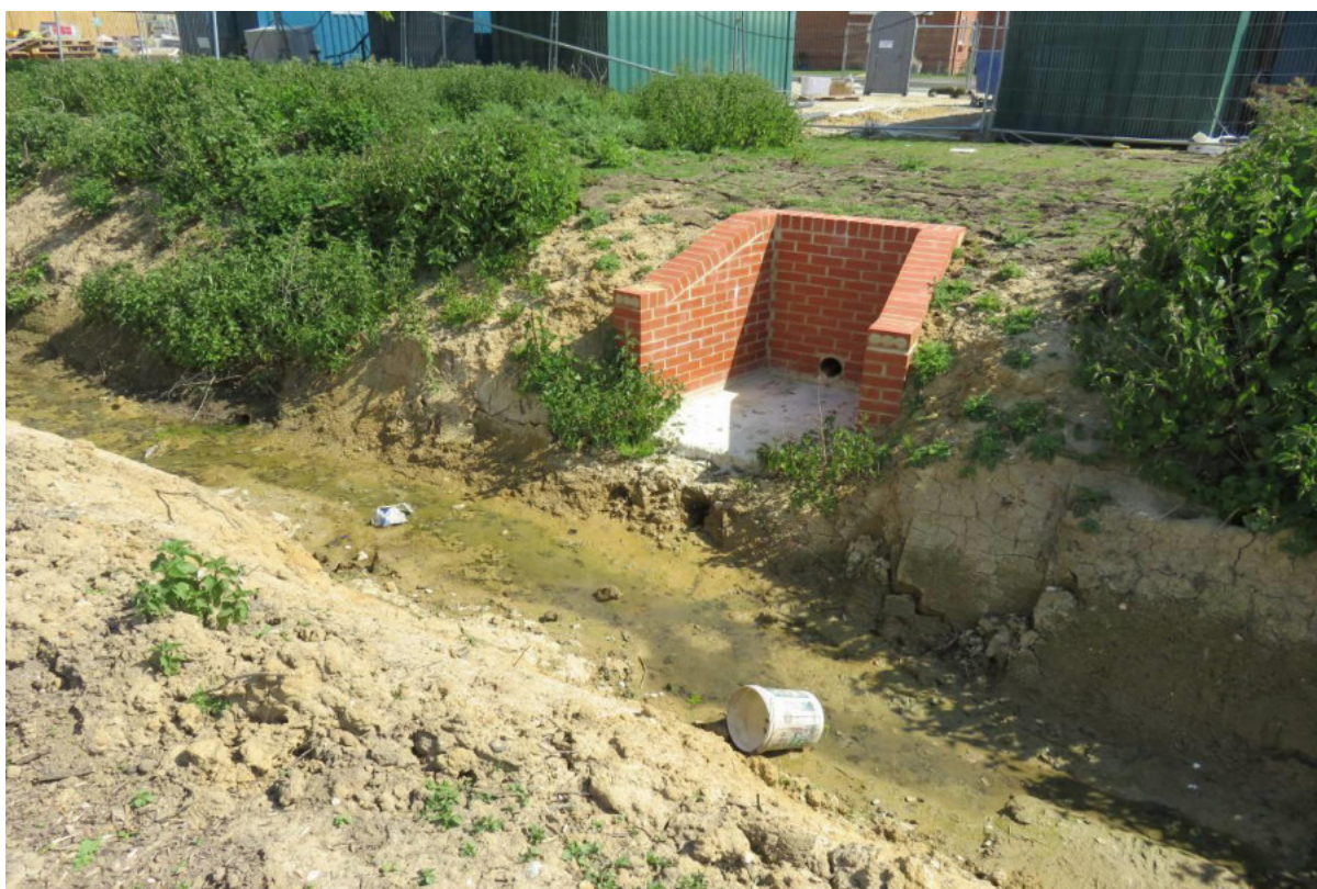
Works to northern boundary watercourse on site and off site to north
