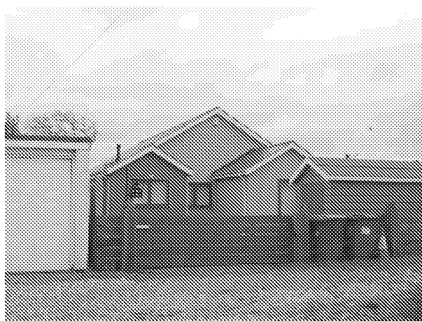
Image 4: Front elevation of No. 75 West Front Road.
