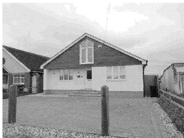
Image 3: Front elevation of No. 80 Harbour Road.
