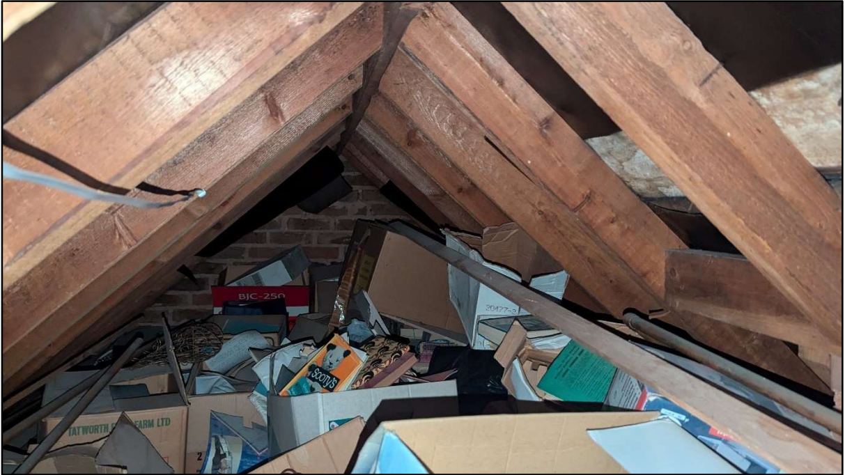
View inside the loft.
