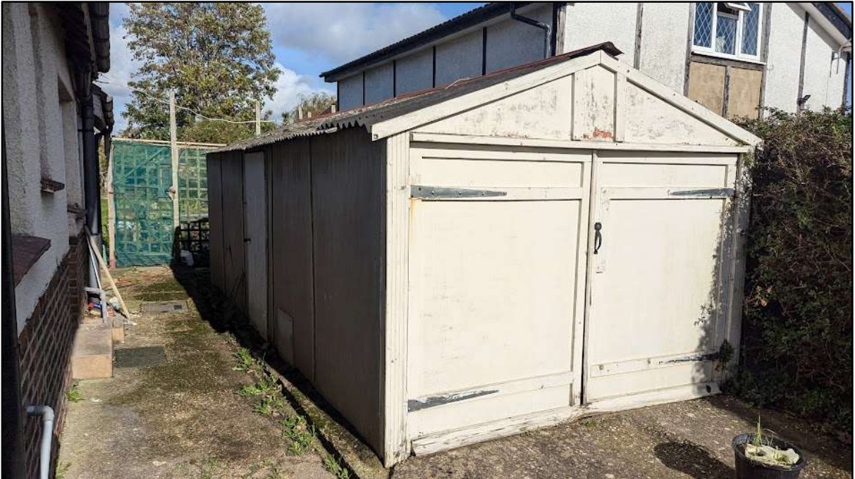
View of the small timber garage.
