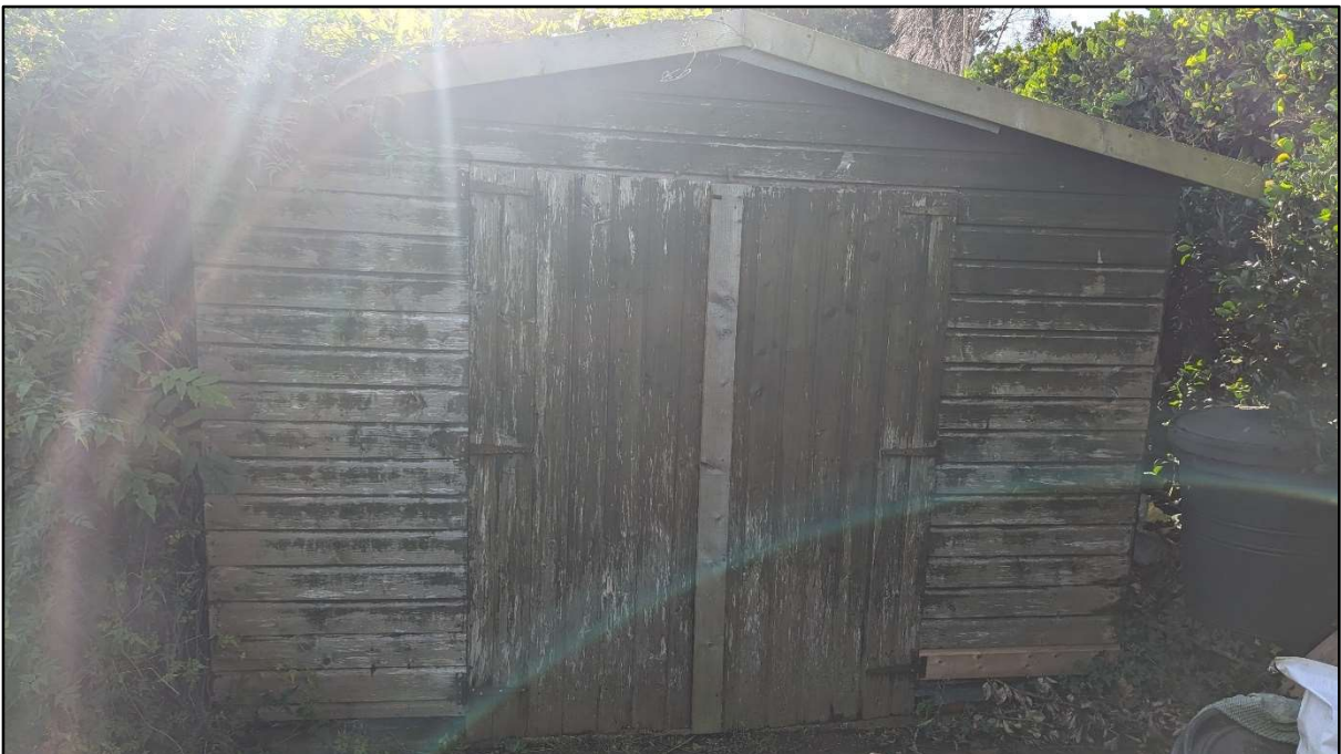
The timber workshop/shed.
