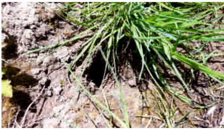
Small burrows seen within the bank, too small to be water voles.
