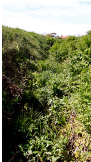
Photo 3. Eastern sections of Ditch which have less water and more vegetation coverage.
