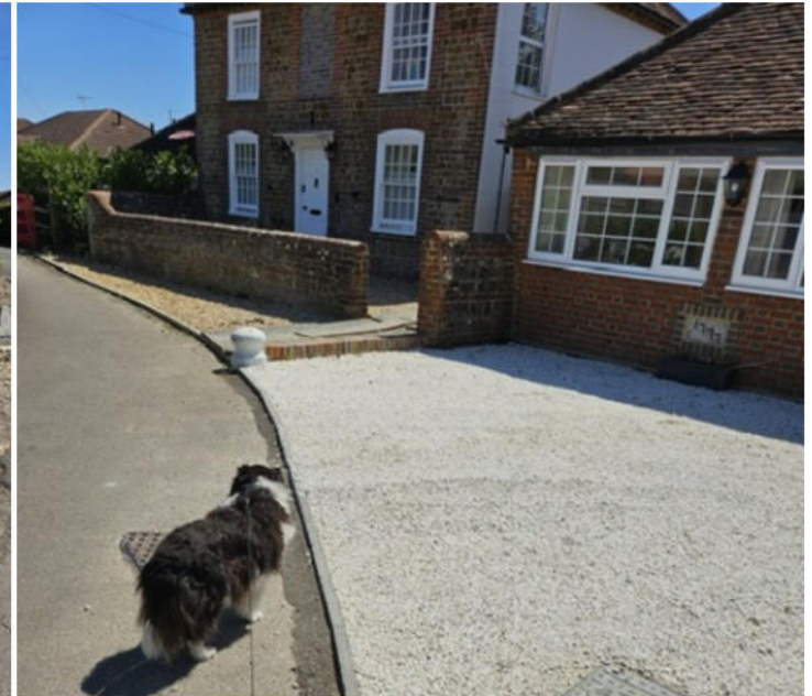
Unsympathetic fenestration in the garage conversion
